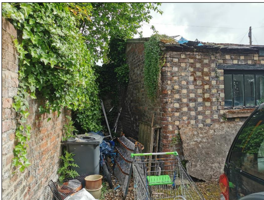
Plate 4 – The garage west facing gable elevation
