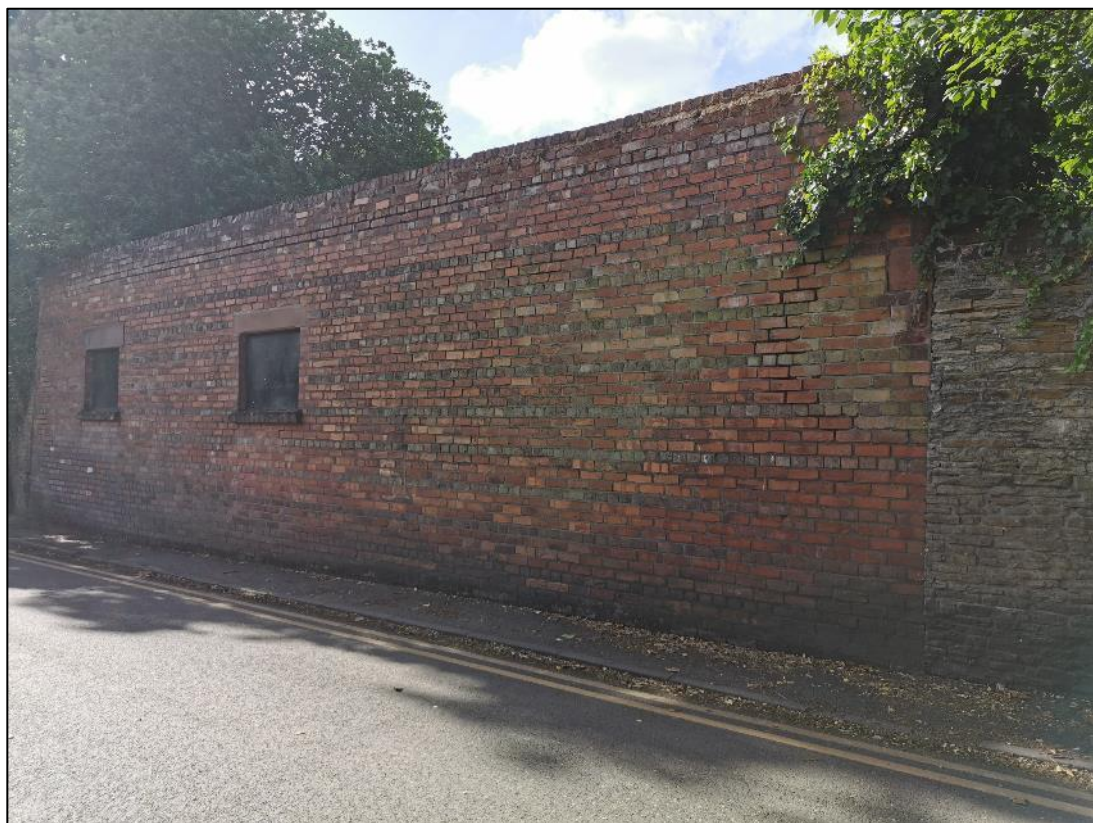
Plate 2 – The garage along the wall in the north of the site, rear, north facing aspect
