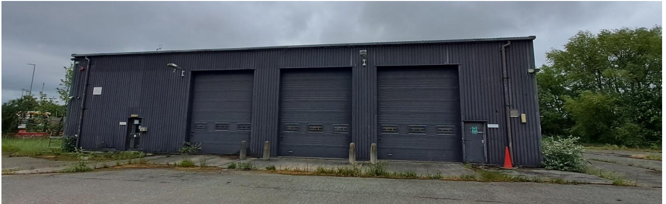
Figure 5: The on-site building B1
