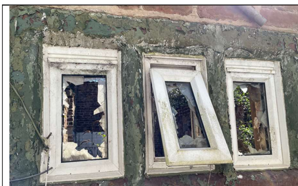
North elevation – an example of the poor condition of the stone and masonry.
