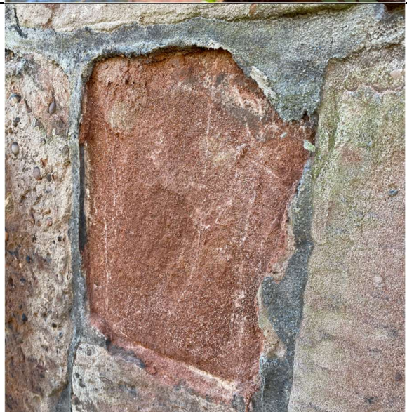
Example of cementitious mortars accelerating the decay of the soft local red sandstone.
