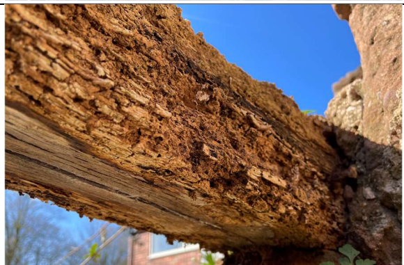
Example photo of the decay of one of the three remaining 'original' timbers.
