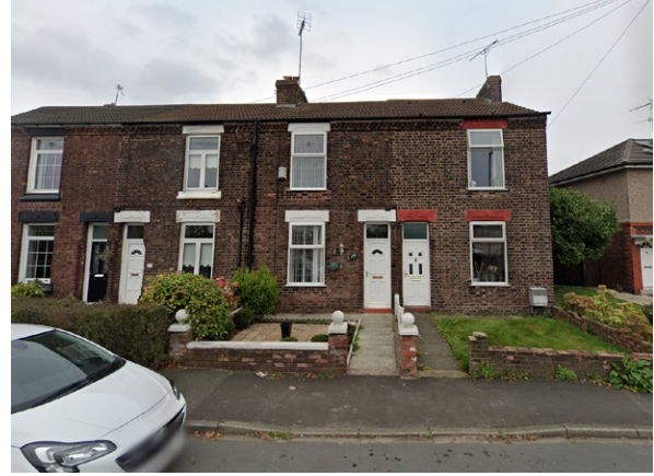
02 - Old Terrace, Hall Lane
