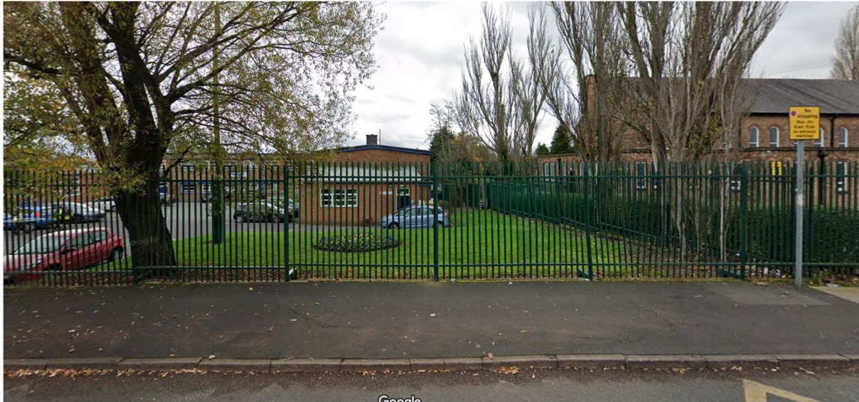
(Existing boundary fencing and evidence of pupils currently needing to walk across the school carpark to access the school)
