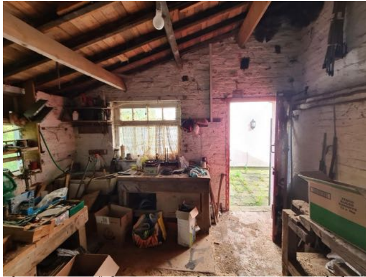
Plate 6- View of the interior to the rear outrigger attached to the 'garage' building. Facing east.
