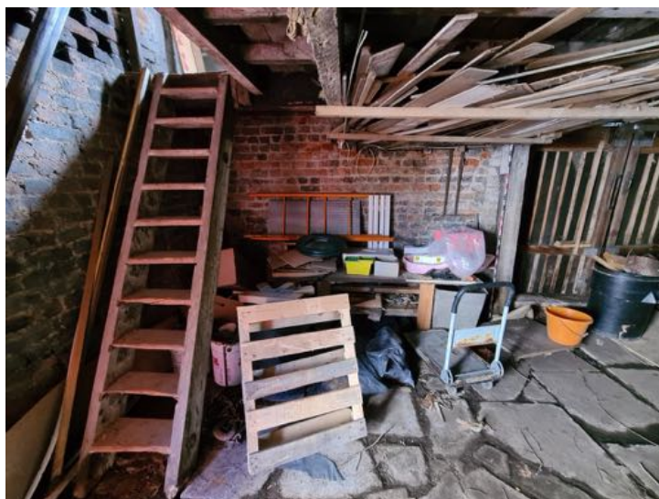
Plate 4- View of the ground floor interior to the 'garage' building with staircase to first floor level. Facing south.
