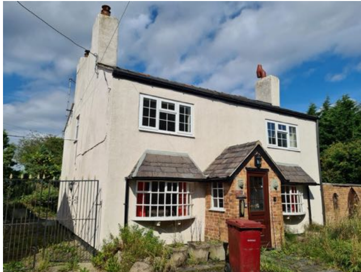
Plate 8- View of the exterior frontage to the main dwelling building. Facing northeast.
