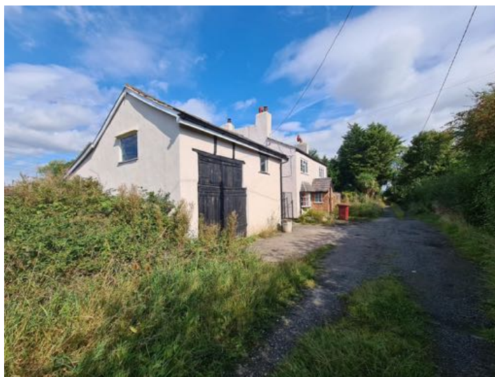
Plate 2 - View of the buildings known as 'Woodlands' fronting on to Lodge Lane. Facing northeast.
