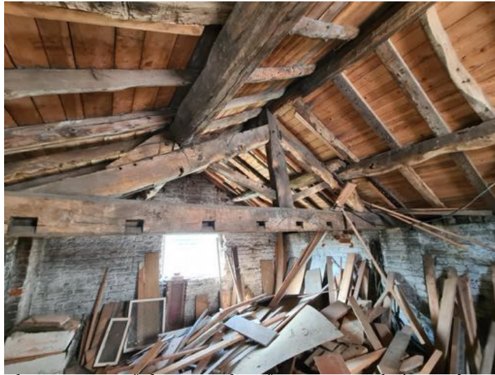
Plate 5- View of the internal roof structure to the 'garage' building at first floor level. Facing west.
