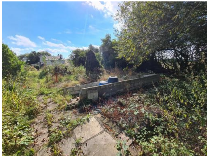
Plate 10- View of the remains to an outbuilding built from concrete blocks at the northern end of the garden area. Facing southwest.
