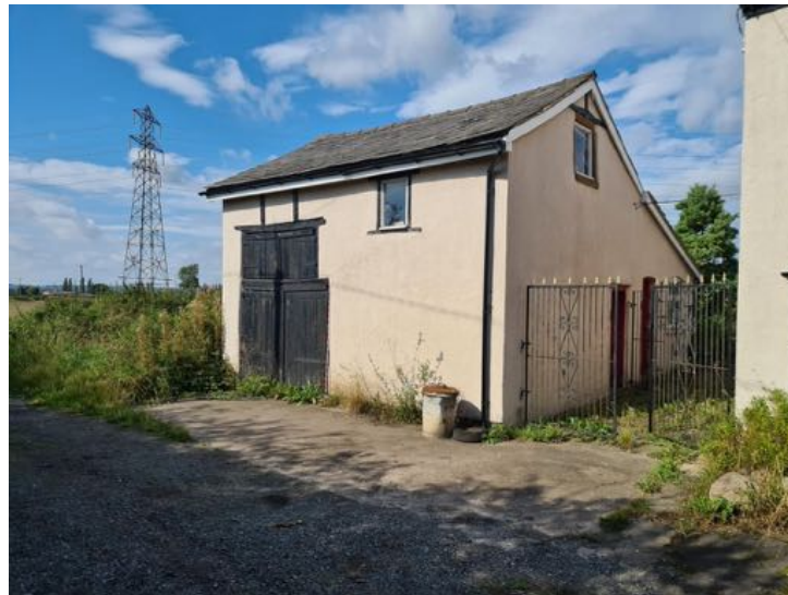
Plate 3- View of the 'garage' building fronting on to Lodge Lane. Facing northwest.
