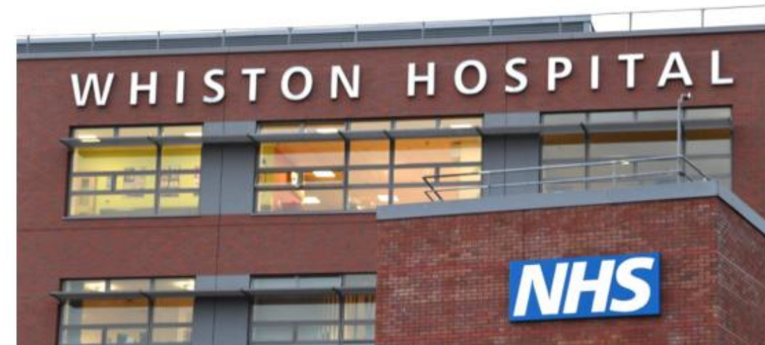
Existing hospital brickwork
