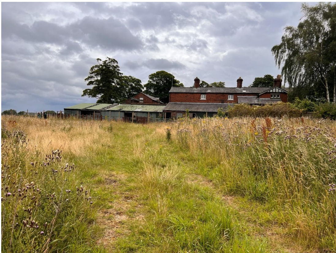
Plate 2: Looking towards Park Farm. The brick upper storey is no earlier than 19 th century and may be later.
