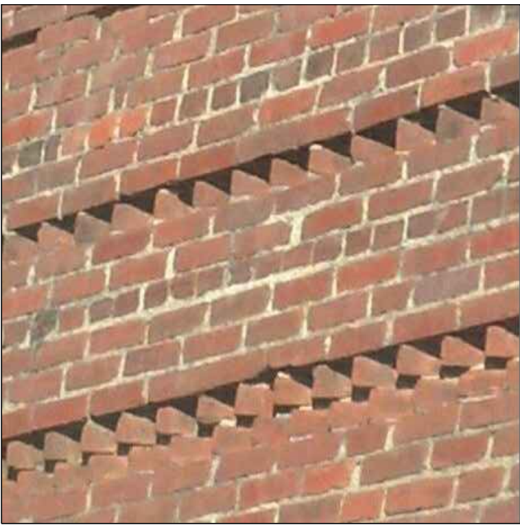
2 Feature Brick Dental Bandcourse Detailing
