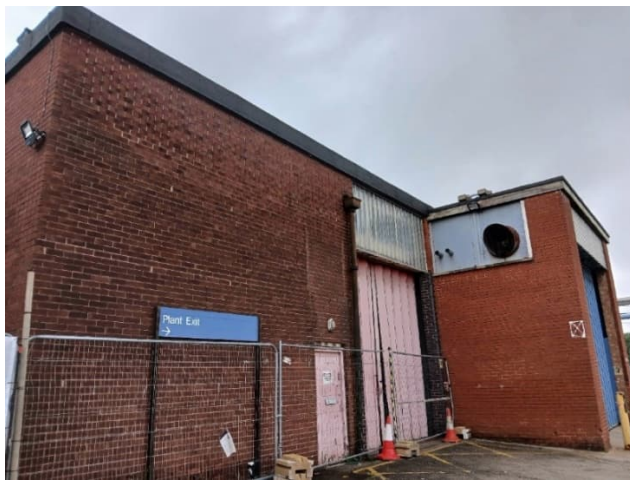
Photograph 3 – B3: Three sets of large shutter doors left open allowing access into building with many potential roost features inside. Small, high gap at end of metal sheeting leading into cavity wall. Three access points into single story section of building, two holes in brickwork into cavity wall, open vent leading into roof cavity.
