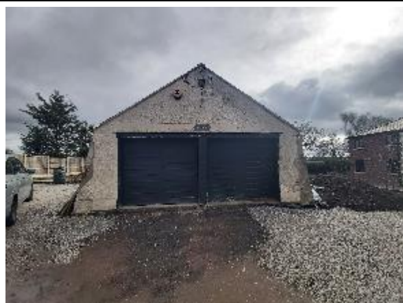
Detached Garage (proposed for demolition) and surrounding bare ground / hardstanding.
