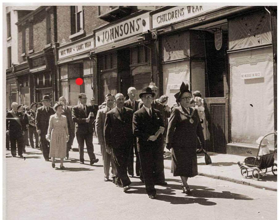
Historic photograph of 25-29 Eccleston Road from 1951
