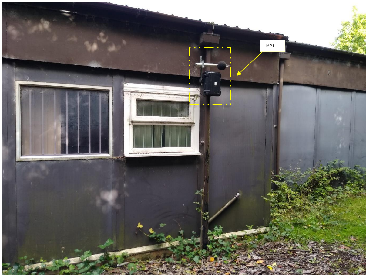
Figure 2.0 – Microphone location located on a drain pipe from the existing development.
