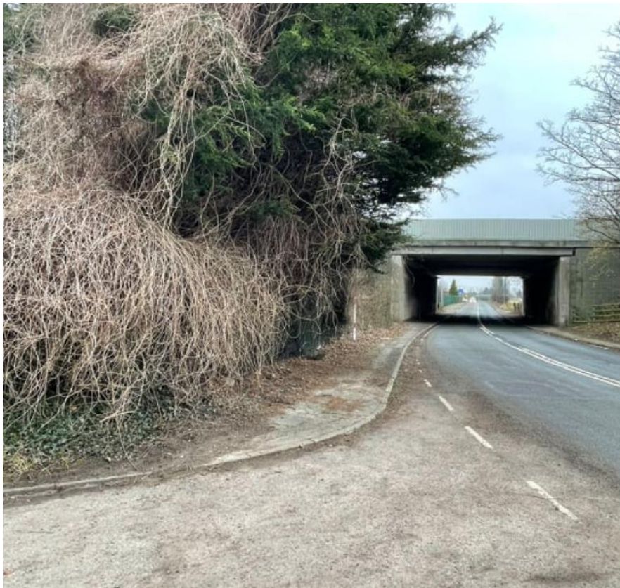
Western site boundary looking south along Lower Road
