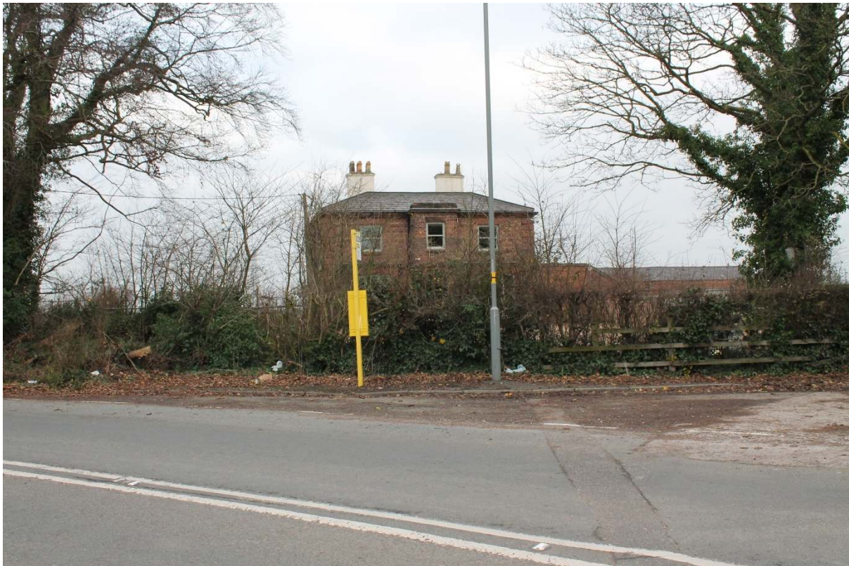
Figure 2.9: Brook House Farm villa
