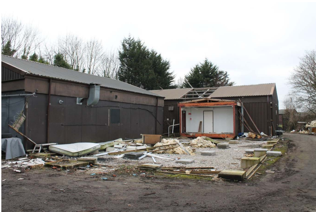
Figure 2.3: Foundations for the northern building
