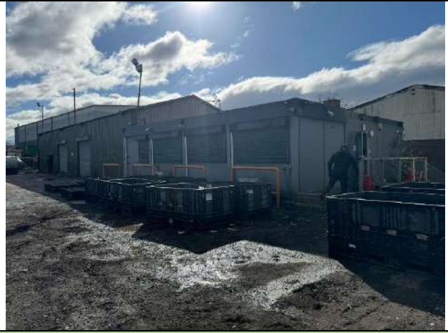
P2: Buildings in the south
