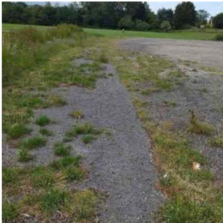
Photo 12: Asphalt surfacing along the eastern car park boundary (photograph taken facing south).
