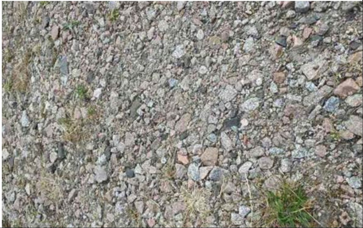
Photo 11: Car park surface composed of fine to coarse gravel of granite and limestone.
