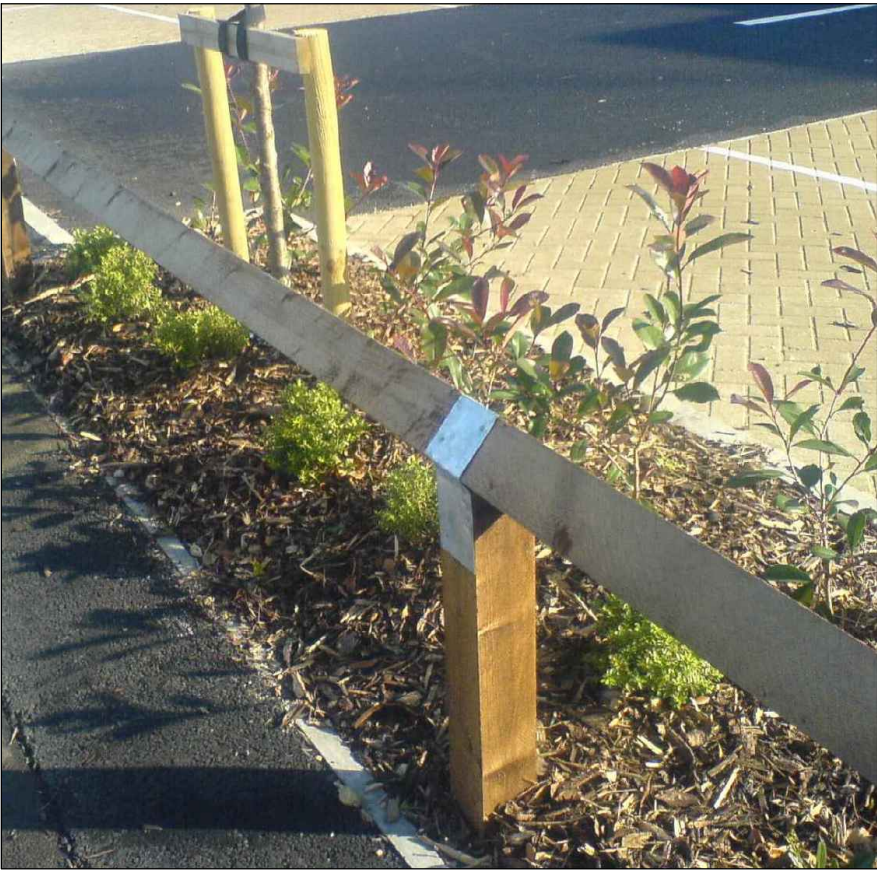
Timber Knee Rail Timber birdsmouth posts, 70 x 70mm, with a top rail 91 x 91mm.
