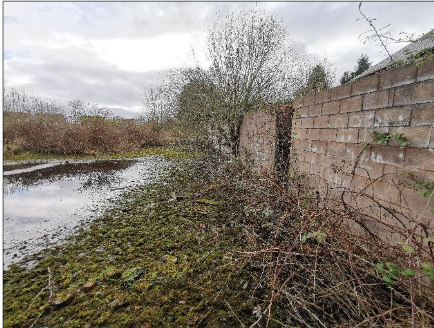
Plate 11 - Area of hardstanding in the north of the site
