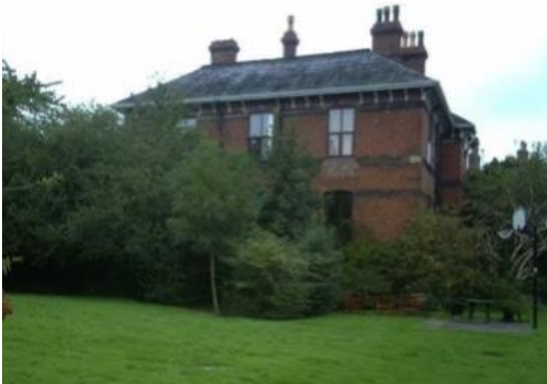
FIGURE 12 ST ANNE'S LOCATED TO THE NORTH OF THE APPLICATION SITE © KDP ARCHITECTS 2019
