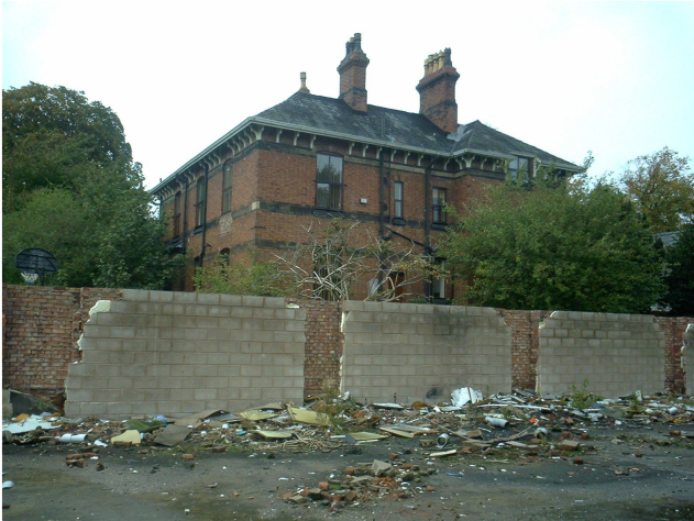
Site View showing remnants of the Sports Hall
