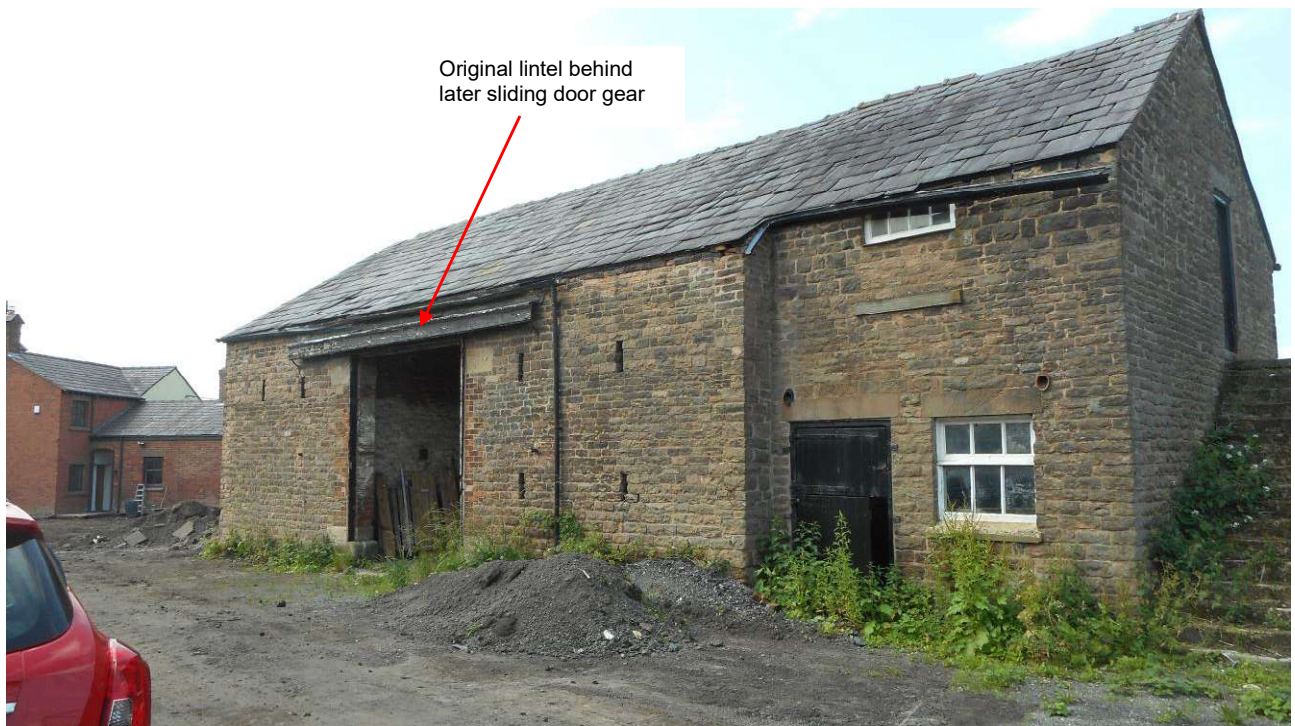
Above: Stone Barn east facing elevation
