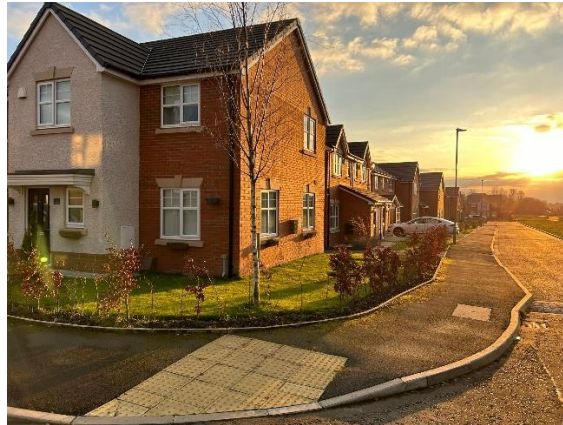
Location of blister paving away from proposed car parking space.
