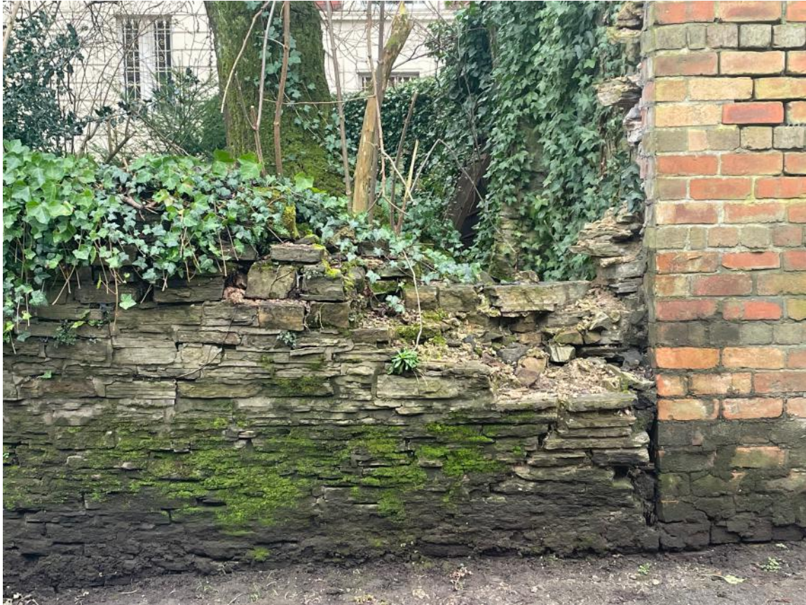
Photo 1: West End of Wall
