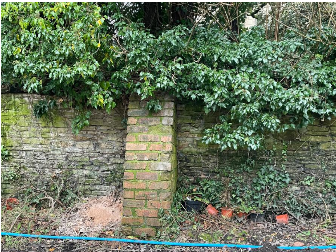
Photo 6: North Side of Wall
