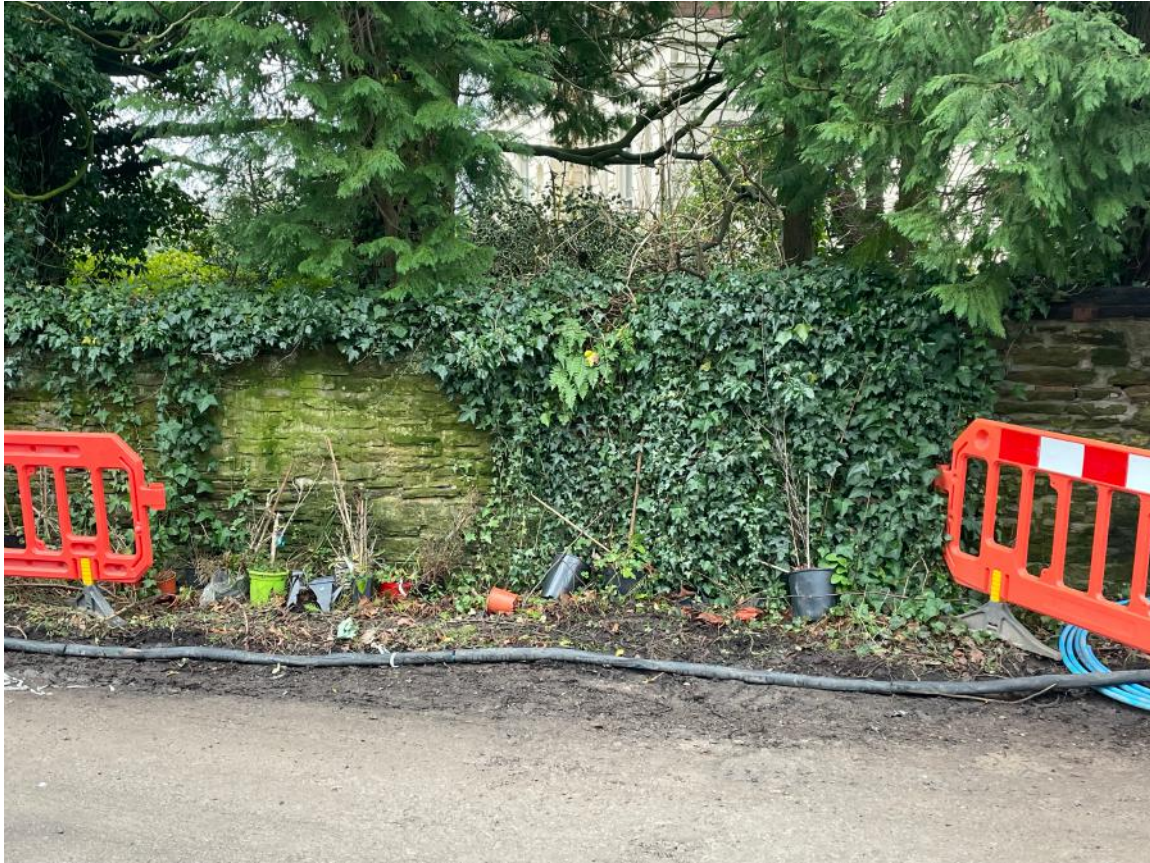
Photo 3: North Side of Wall
