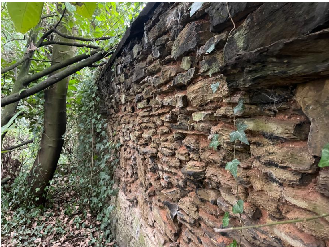
Photo 8: South Side of High Wall in Garden
