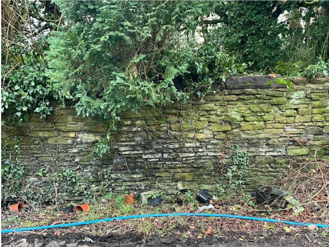
Photo 5: North Side of Wall
