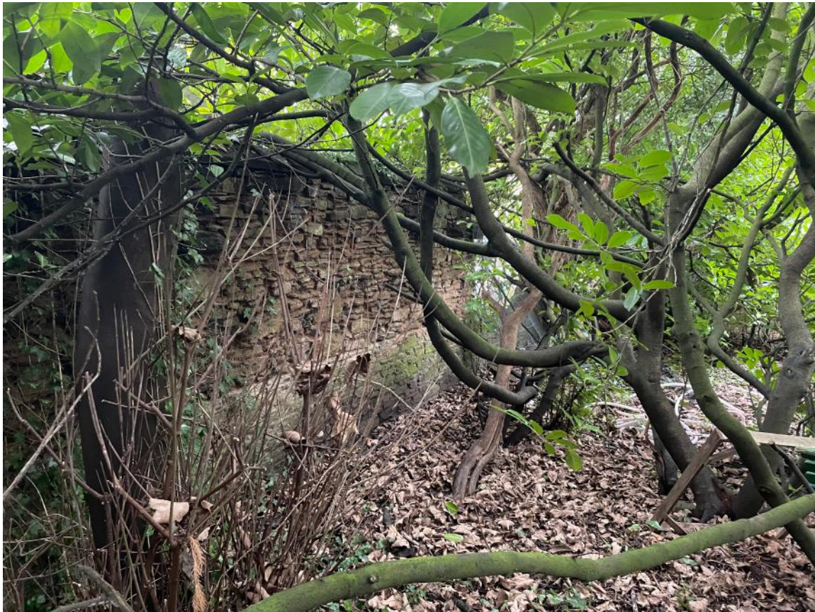
Photo 9: South Side of High Wall in Garden
