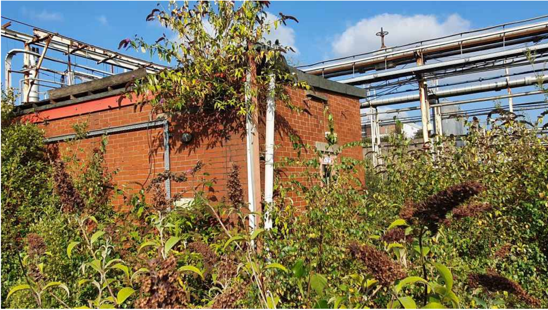
03 Building 18 Existing - Photograph of South/West Elevation 1:2000 @ A1
