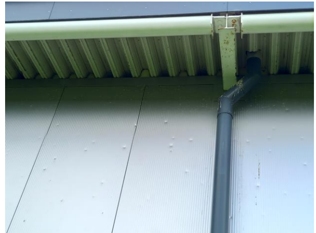
Photograph 16 – Halewood leisure centre potential bat roost feature (PRF), gaps where roofing sheets join the building.
