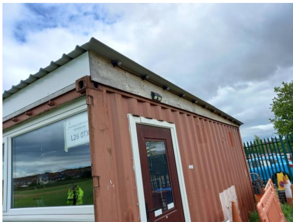
Photograph 21 – Building 5, PRF. Gaps located under roofing sheets.
