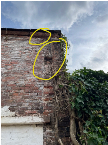
Install New Bricks To Missing Areas
