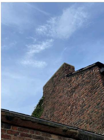
Rebuild Chimney Stack
