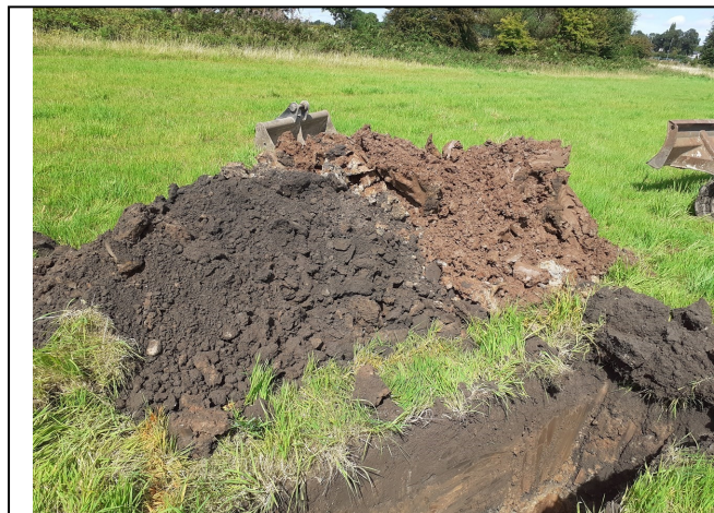
Trial Pit 112 Spoil
