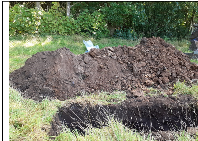
Trial Pit 109 Spoil
