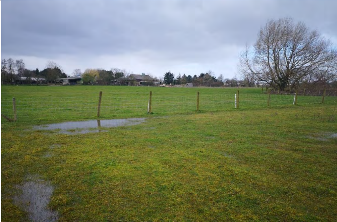
PLATE 5 POOR DRAINAGE WITHIN CATTLE GRAZING FIELD (WEST)
