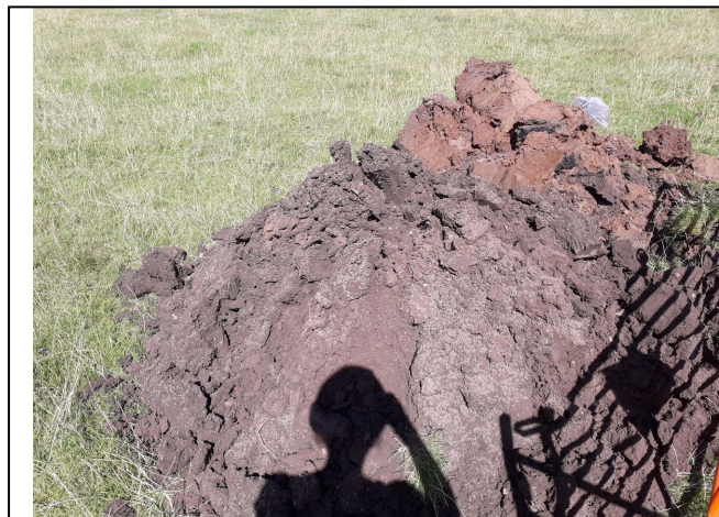
Trial Pit 108/ Soakaway 106 Spoil
