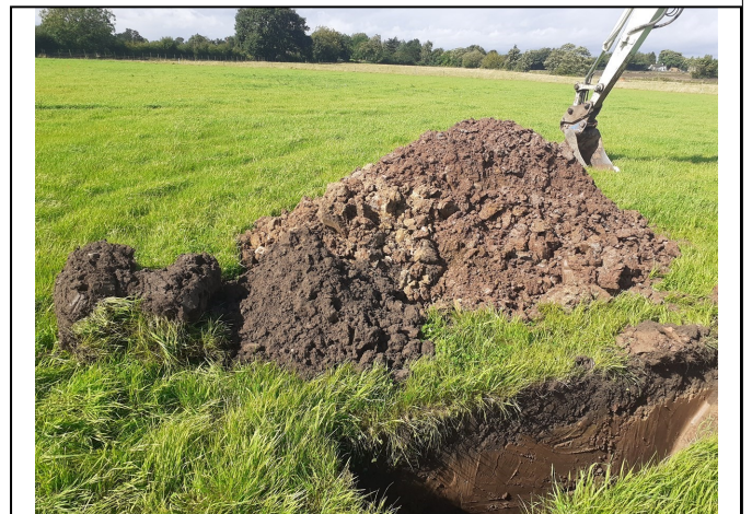
Trial Pit 125 Spoil
