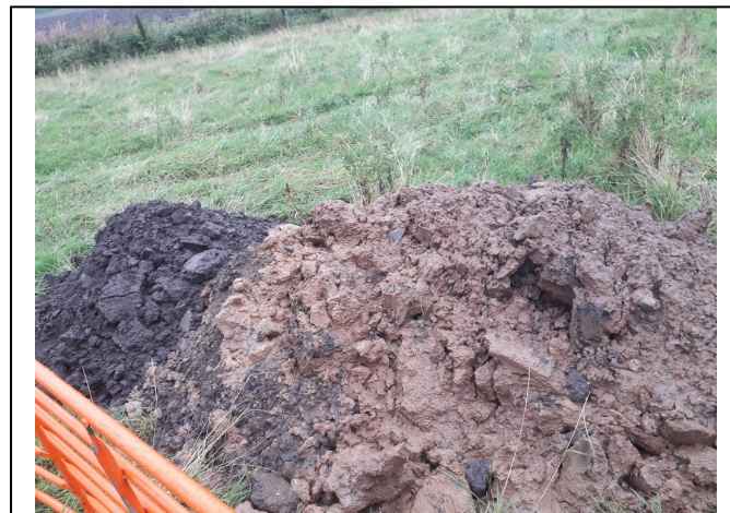
Trial Pit 105/ Soakaway 103 Spoil
