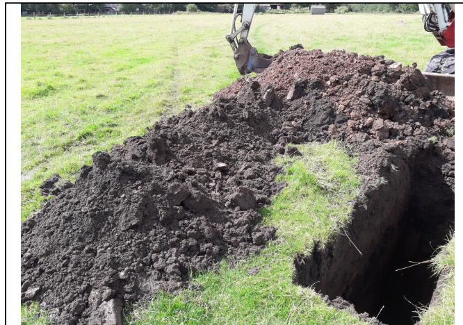
Trial Pit 137 Spoil
