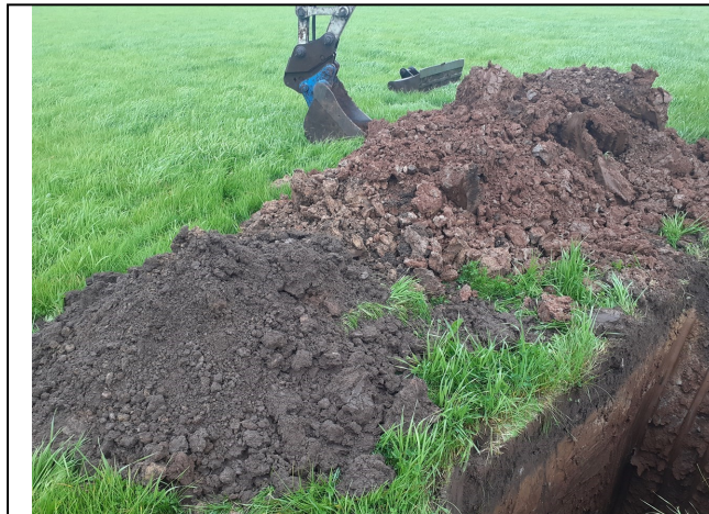
Trial Pit 120 Spoil
