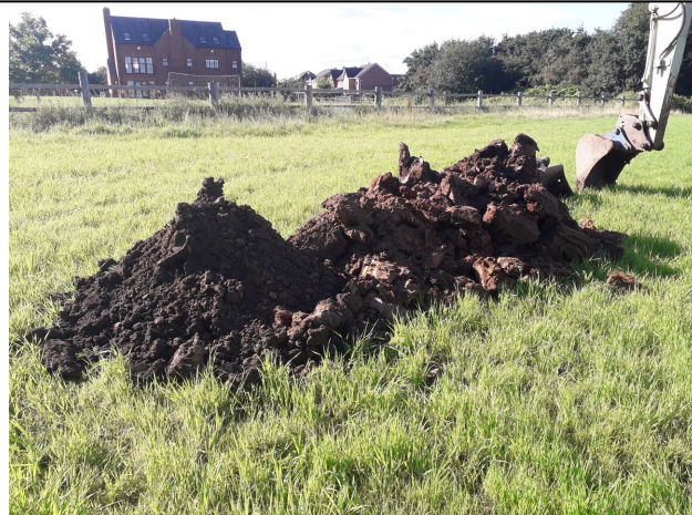
Trial Pit 101/ Soakaway 101 Spoil
