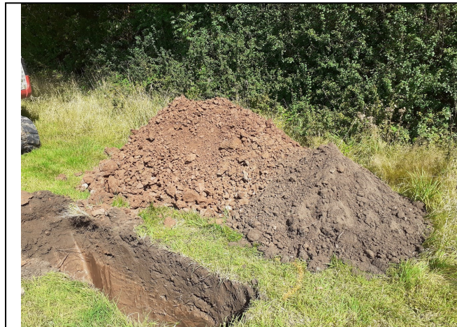
Trial Pit 111 Spoil
