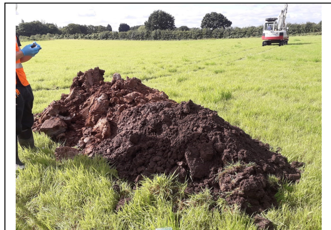
Trial Pit 104/ Soakaway 102 Spoil
