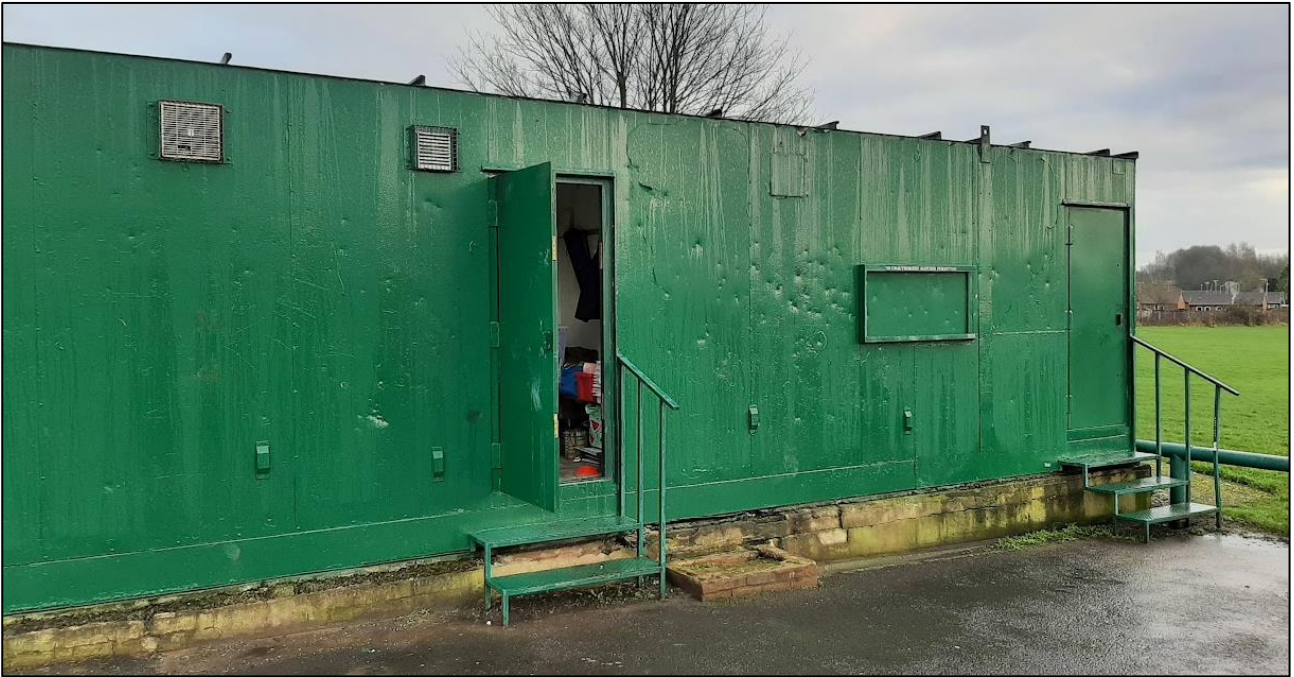
Figure 9: Shipping containers southern elevation
