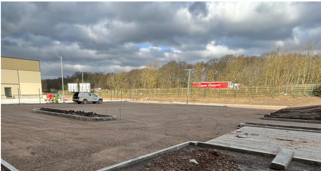
Photo of existing site looking north towards M57
