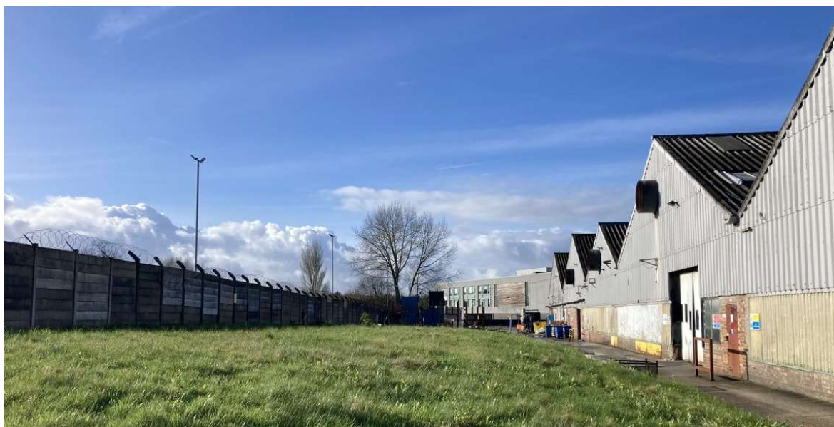
PLATE 1 WESTERN BOUNDARY OF FACTORY BUILDING (FACING SOUTH)
