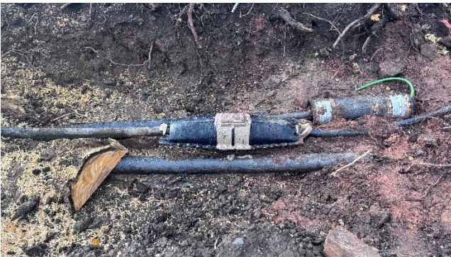
Plate 9 View showing repaired electrical cable in the southern area of the site
