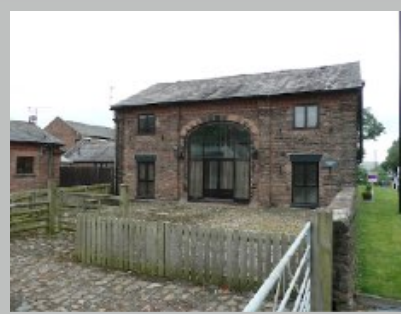
Plate 29. Former farm building on School Lane
