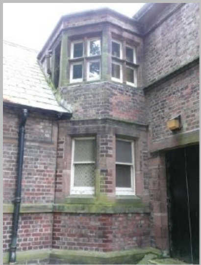
Plate 14. Canted link at rear
