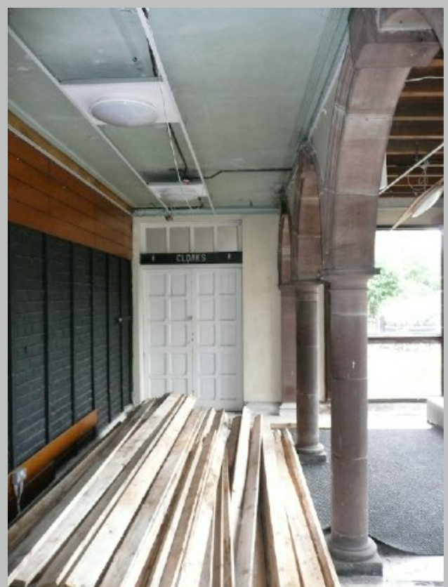
Plate 5. Front arcade, currently inside the porch
