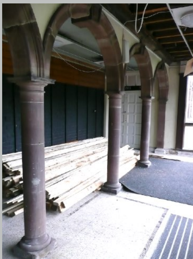
Plate 4. Front arcade, currently inside the porch
