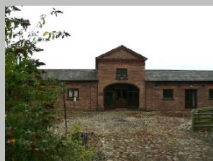
Plate 28. Former farm building on School Lane
