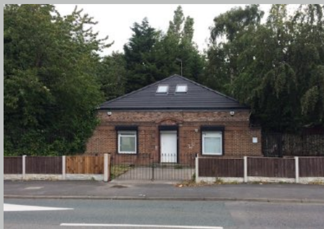
Plate 44. Estate building/lodge, disfigured by alterations
