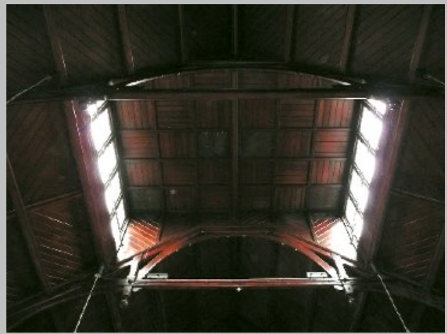
Plate 19. Lantern and trusses
