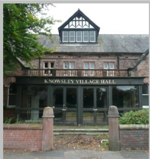
Plate 17. Central entrance on School Lane
