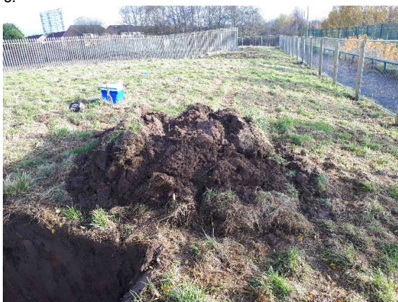
Trial Pit 2 – Arisings 1
