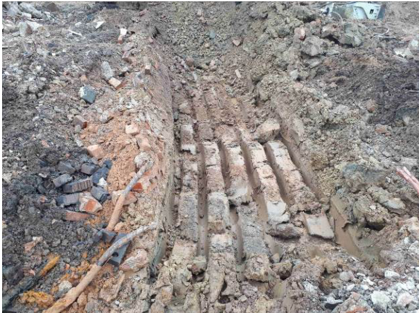
04.04.18 – Post-electricity substation slab removal – underlying natural soils.
