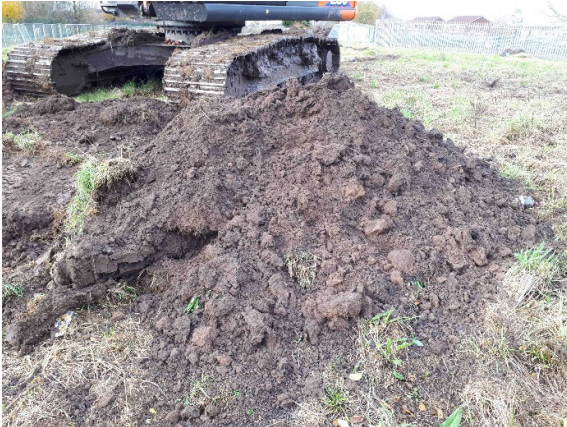
Trial Pit 3 – Arisings 1
