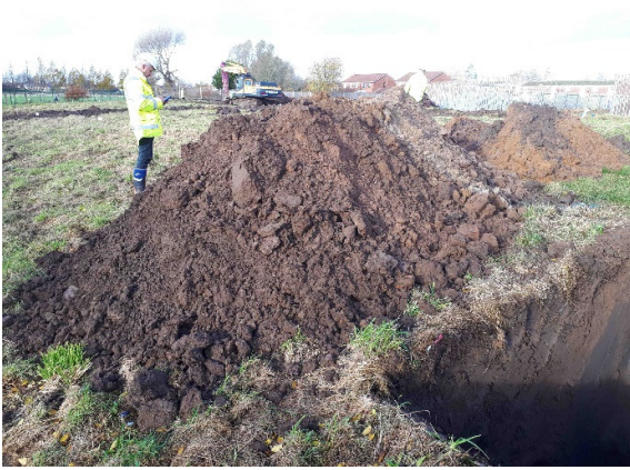
Trial Pit 2 – Arisings 2
