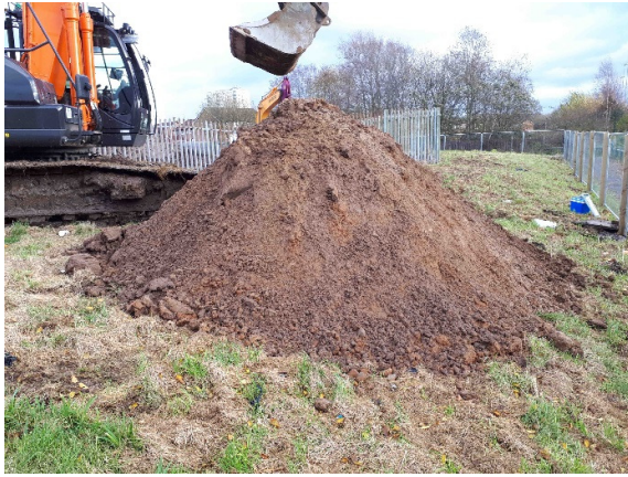
Trial Pit 3 – Arisings 3
