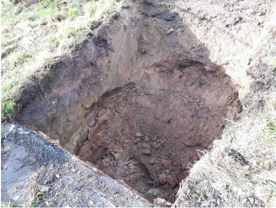
Trial Pit 3 – View of pit 1
