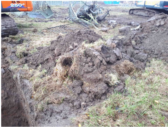
Trial Pit 4 – Arisings 1
