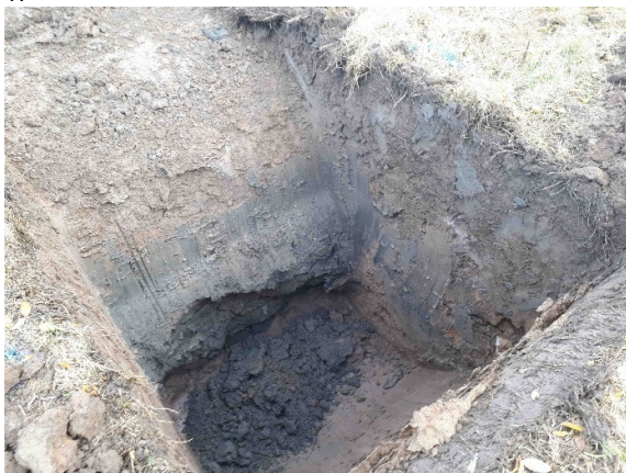
Trial Pit 1 – View of pit
