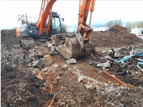
04.04.18 – Electricity substation slab removal.
