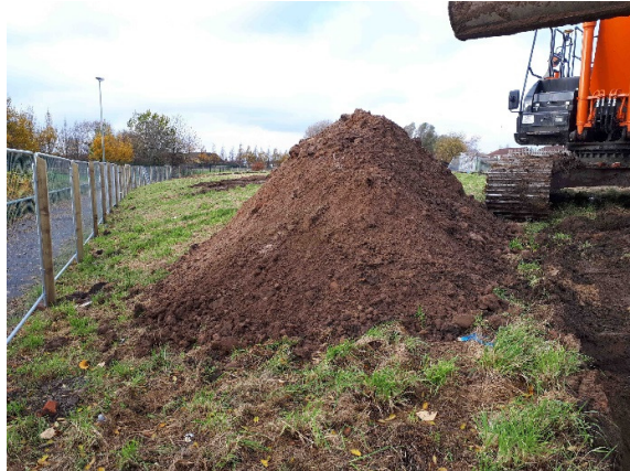
Trial Pit 3 – Arisings 2
