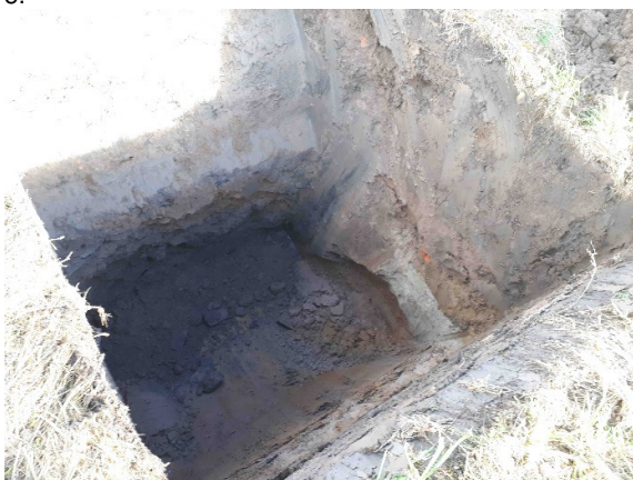
Trial Pit 2 – View of pit
