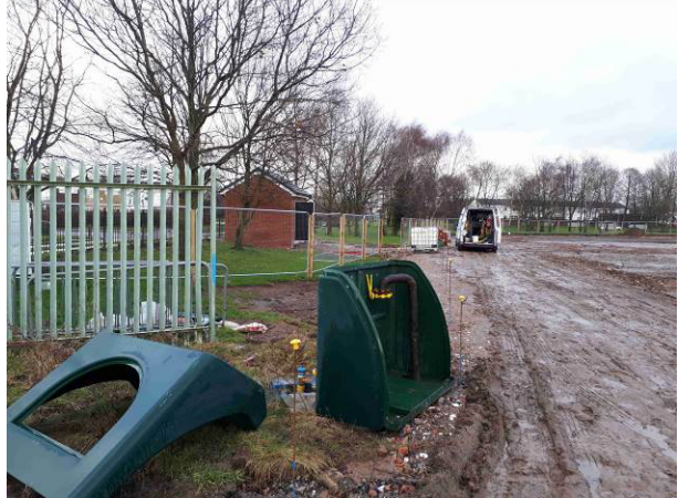
15.01.18 – Construction of electricity substation located along centre of northwest boundary complete.
