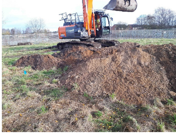
Trial Pit 2 – Arisings 3
