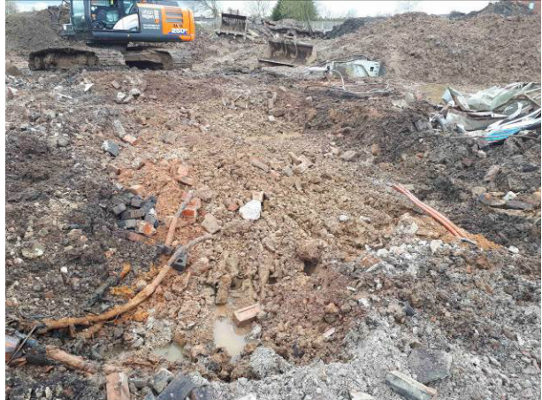
04.04.18 – Post-electricity substation slab removal – underlying made ground.
