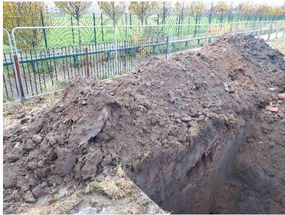
Trial Pit 4 – Arisings 2
