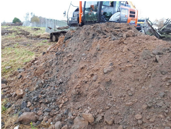
Trial Pit 4 – Arisings 3
