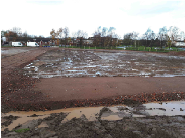
23.11.17 – Laid crushed aggregate in road positions in centre-north of site.
