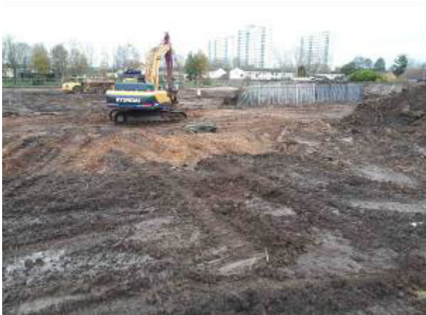
14.11.17 – Turnover of made ground soils with excavator in centre-west part of site.
