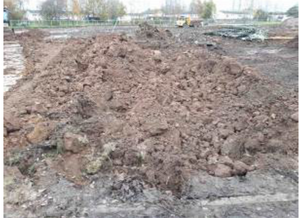
14.11.17 – Turned over made ground soils in centre-west part of site prior to recompaction.
