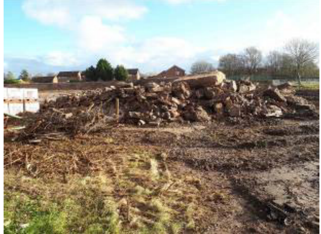
23.11.17 – Stockpile of hardstanding in centre of site recovered from turnover of made ground soils in central parts of site.
