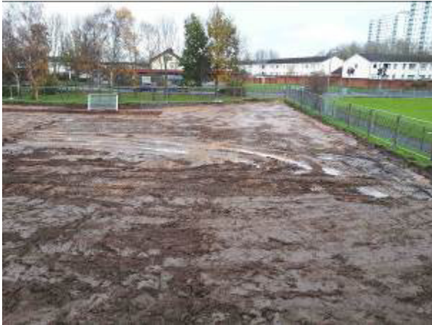
14.11.17 –View of northeast corner of site; vegetation and topsoil strip completed prior to inspection.
