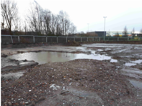
15.01.18 – Topsoil / vegetation strip and turnover of soils completed in southern part of site; placed 6F2 aggregate for basal road construction in south east visible in foreground.
