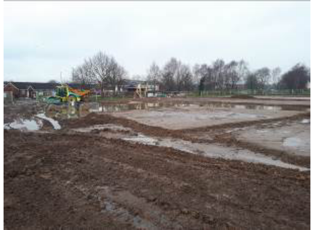
18.12.17 – Crushed aggregate placed in plot footprints in central/northern parts of the site (1/3).
