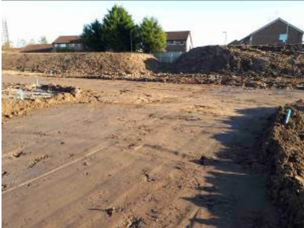
30.11.17 – Footprints of roads dug out in central / eastern parts of site (1/3).
