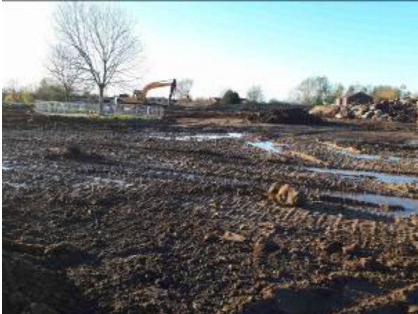
30.11.17 – Turnover of soils in in centre-south of site with excavator (in far distance).
