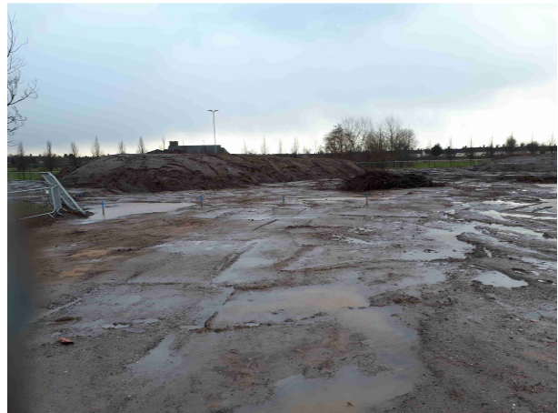
15.01.18 – Topsoil stockpile in southwest of site.
