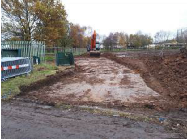
14.11.17 – Digging out of road footprint with excavator along northwest boundary.
