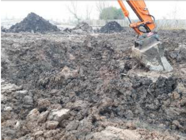
18.12.17 – Turnover of soils and excavation of peat in the northern part of the western section of site; peat stockpiles visible in background.
