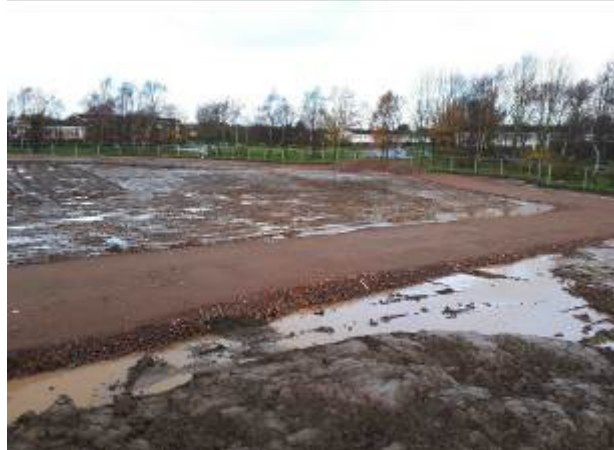
23.11.17 – Laid crushed aggregate in road positions in north of site.
