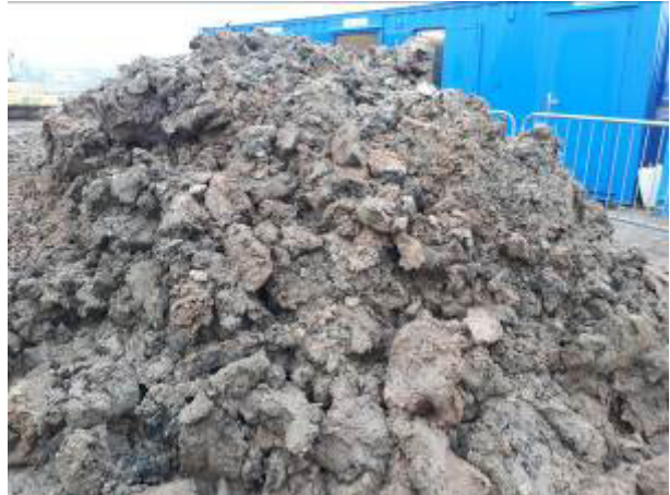
18.12.17 – Clay / peat stockpile excavated from the northern part of the western section of site.
