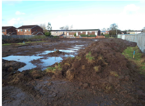
23.11.17 - Vegetation and topsoil strip in the northern part of the western section of site completed prior to inspection.
