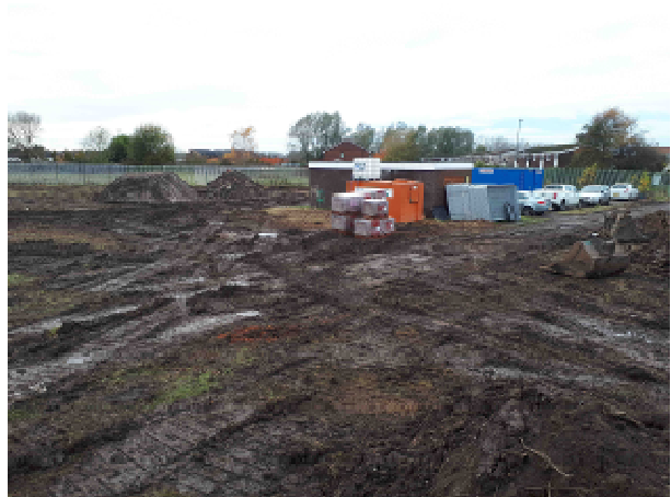
14.11.17 – View west from centre of site; electricity substation visible.
