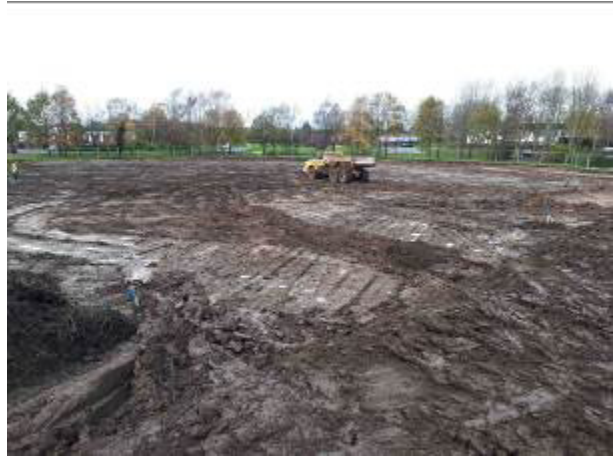
14.11.17 –View northwest across site from northern part of southeast boundary; vegetation and topsoil strip completed prior to inspection.
