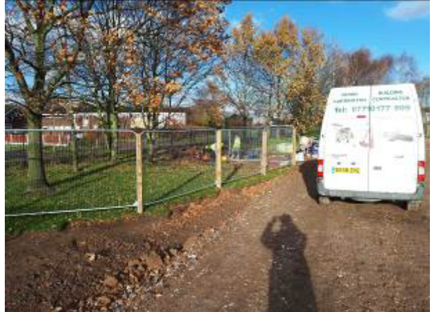
23.11.17 – Construction of electricity substation located along centre of northwest boundary in progress.
