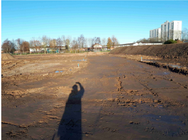
30.11.17 – Footprints of roads dug out in central / eastern parts of site (3/3).
