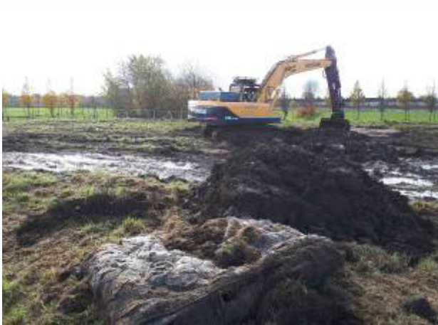
23.11.17 - Vegetation and topsoil strip in the central part of the western section of site.
