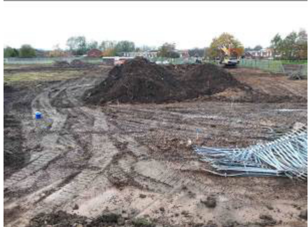
14.11.17 –View west across site from north of southeast boundary; vegetation and topsoil strip completed prior to inspection and stockpile of stripped vegetation visible.
