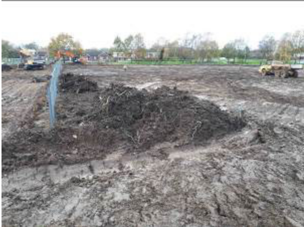
14.11.17 –View west-northwest across site from northern part of southeast boundary; vegetation and topsoil strip completed prior to inspection and small stockpiles of stripped vegetation visible.
