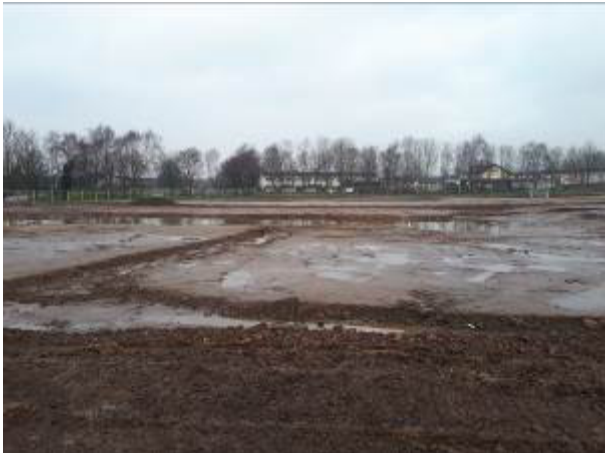
18.12.17 – Crushed aggregate placed in plot footprints in central/northern parts of the site (2/3).
