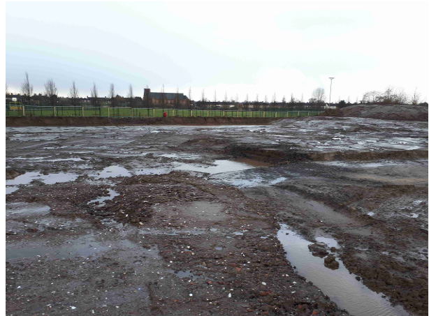
15.01.18 – Topsoil / vegetation strip and turnover of soils completed in the central part of the western section of site; placed 6F2 aggregate for basal road construction in south east visible in foreground.
