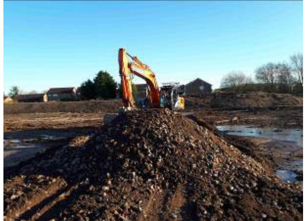
30.11.17 – Laying crushed aggregate in road positions in centre of site with excavator.
