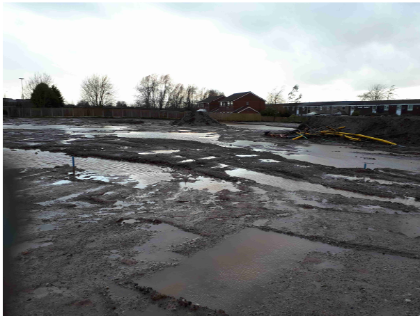
15.01.18 – Topsoil / vegetation strip and turnover of soils completed in in the northern part of the western section of site; peat stockpiles visible.
