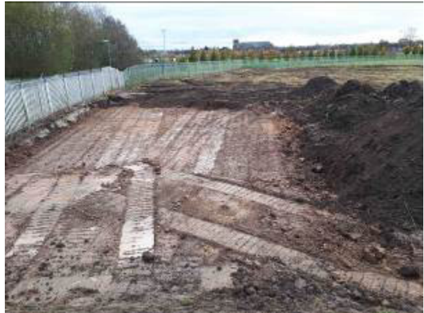
14.11.17 – View of southernmost part of the site including parts of the southeast and southern boundaries; extent of vegetation / topsoil strip visible.
