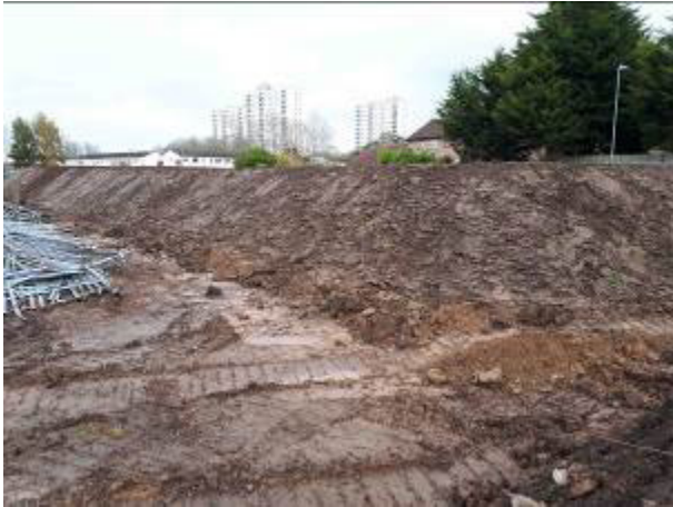
14.11.17 – Topsoil stockpile positioned long southeast boundary, stripped from northern, greenfield parts of site.
