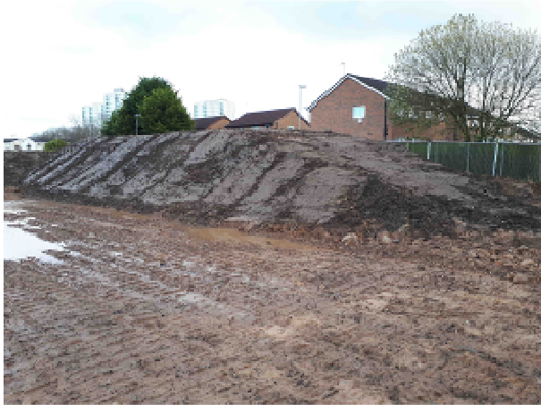
23.11.17 – Stockpile of consolidated stripped vegetation positioned along southeast boundary.
