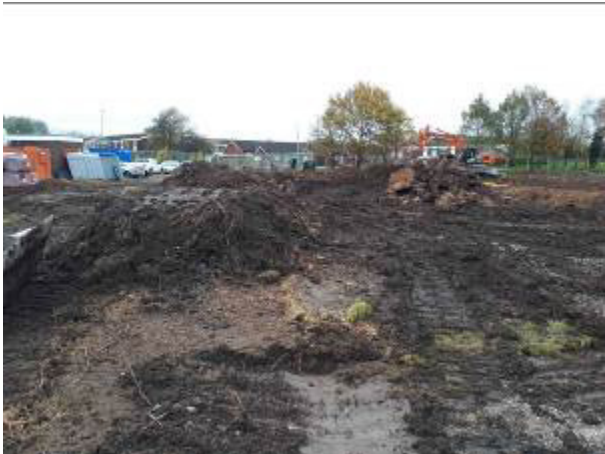
14.11.17 – View west-northwest from centre of site; small stockpiles of stripped vegetation and recovered hardstanding visible following turnover of made ground soils in area.
