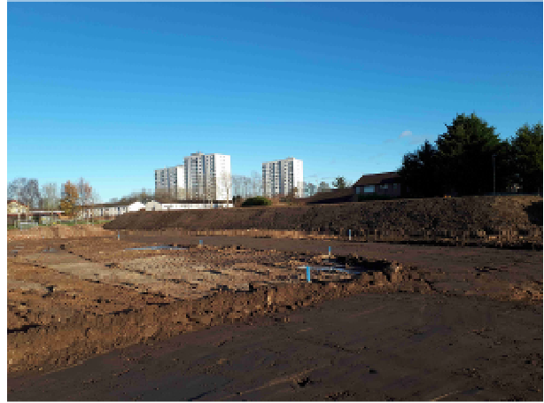
30.11.17 – Footprints of roads dug out in central / eastern parts of site (2/3).
