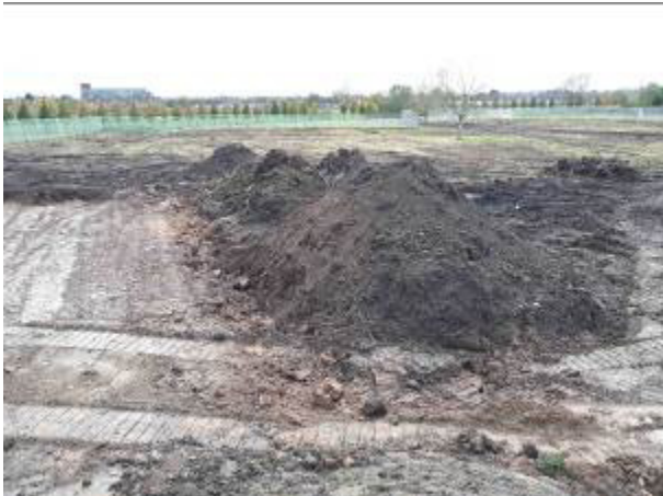
14.11.17 –View west across site from centre of southeast boundary; extent of vegetation / topsoil strip and stockpile of stripped vegetation visible.
