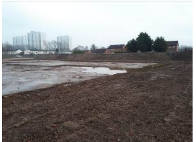
18.12.17 – Crushed aggregate placed in plot footprints in central/northern parts of the site (3/3).
