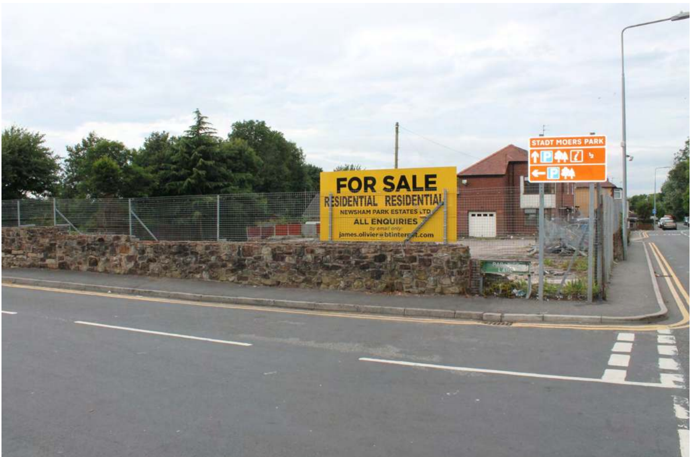
Figure 2.2: Mix of fencing and sandstone/brick walls to Paradise Lane and Greenes Road
