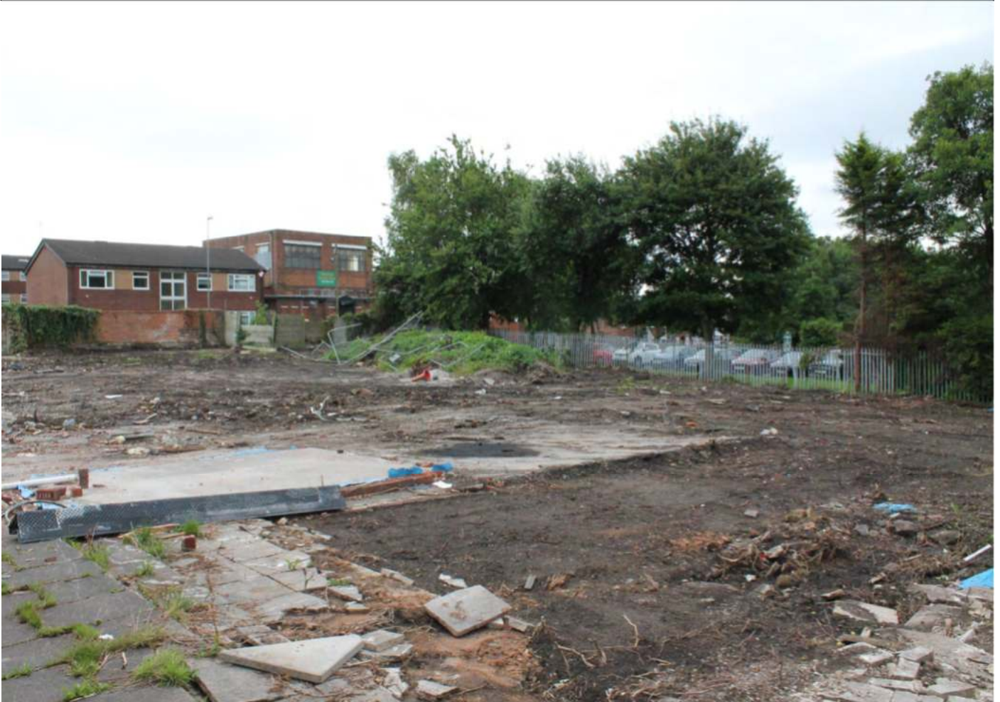
Figure 2.1: Application site looking southeast from rear of 35 Greenes Road
