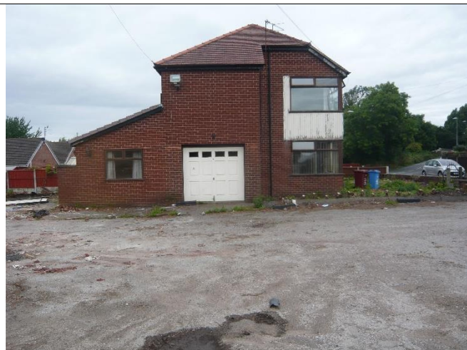
Photo 2: Hard-standing and existing residential property adjacent to western site boundary
