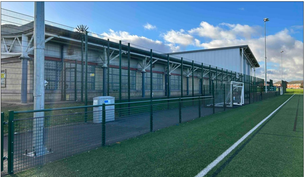
1.1m high crowd barrier and 4.5m high weldmesh fence, looking along the southern length of the AGP hardstanding
