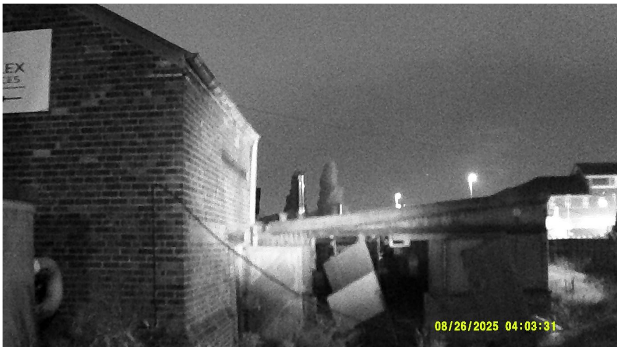
Photograph 10 – Infrared image taken of the northeastern aspect of Building 1 at the darkest point of the survey at 04:03 on 26 th August 2025.
