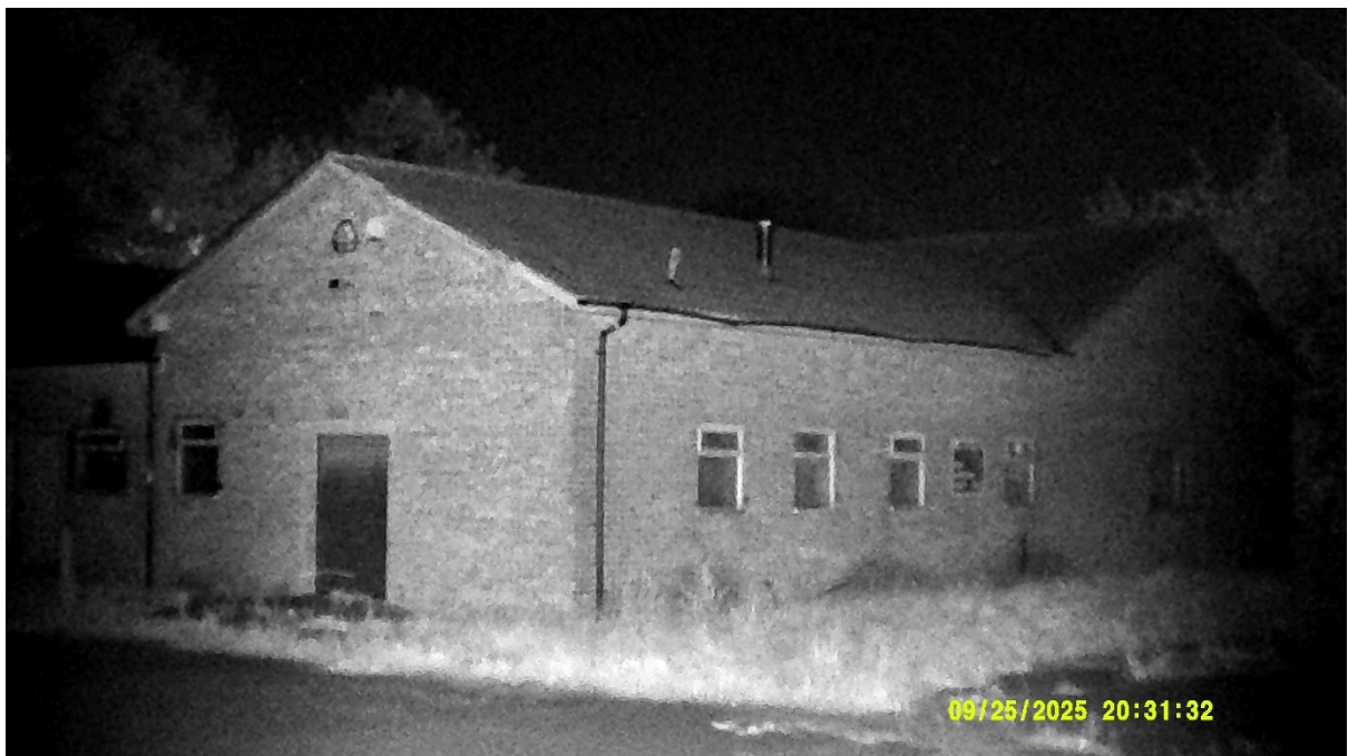
Photograph 16 – Infrared image taken of the northwestern aspect of Building 7 at the darkest point of the survey at 20:31 on 25 th September 2025.
