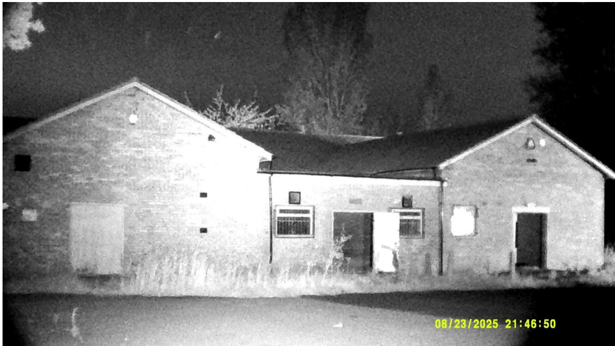
Photograph 5 – Infrared image taken of the aspect of Building at the darkest point of the survey at on.
