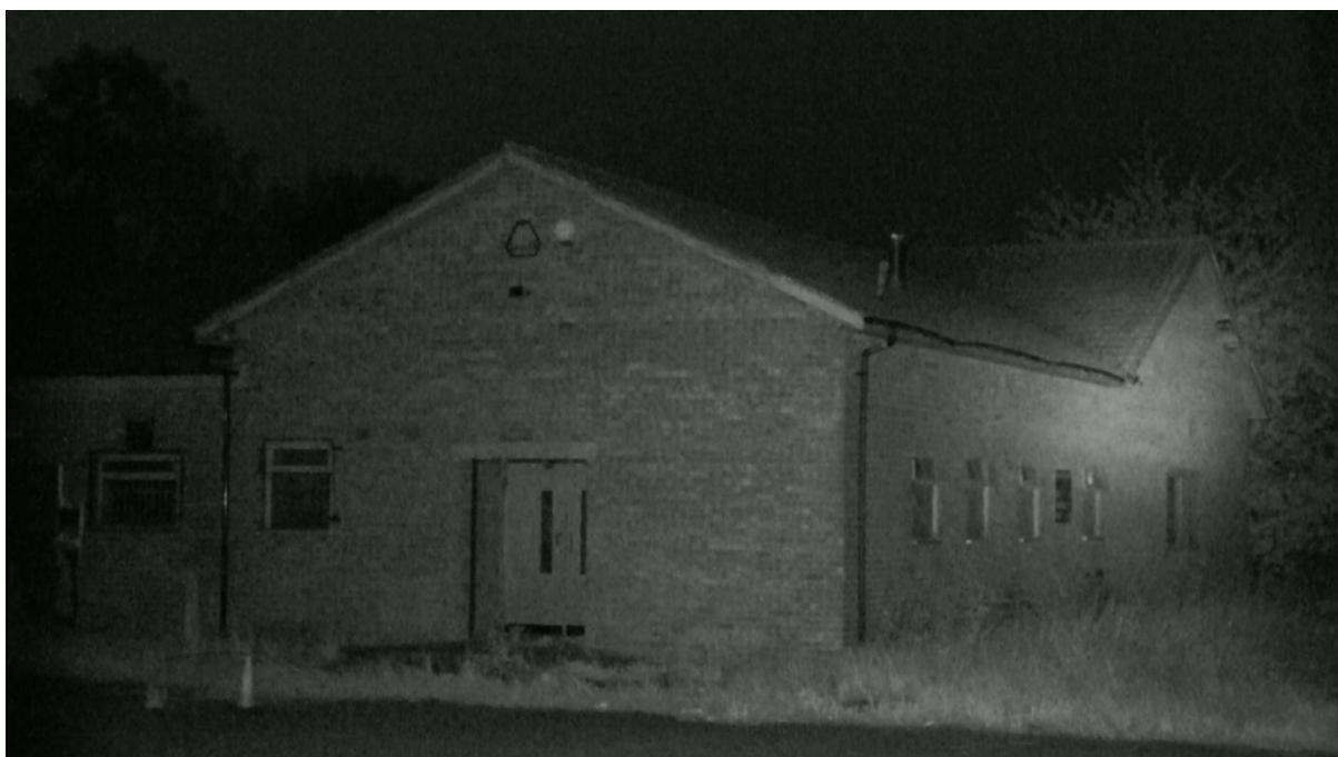
Photograph 4— Infrared image taken of the northwestern aspect of Building 7 at the darkest point of the survey at on.
