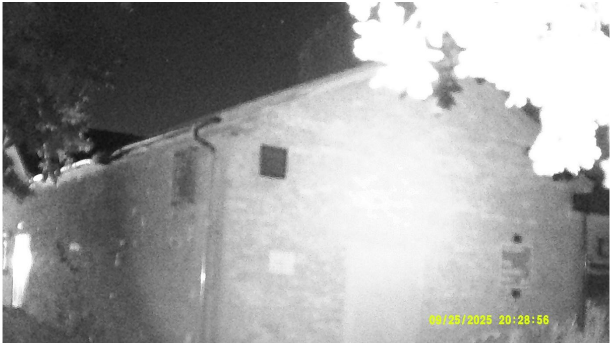
Photograph 15 – Infrared image taken of the northeastern aspect of Building 7 at the darkest point of the survey at 20:28 on 25 th September 2025.
