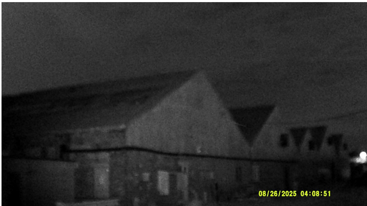
Photograph 6 – Infrared image taken of the aspect of the eastern aspect of Building 1 at the darkest point of the survey at 04:08 on 26 th August 2025.
