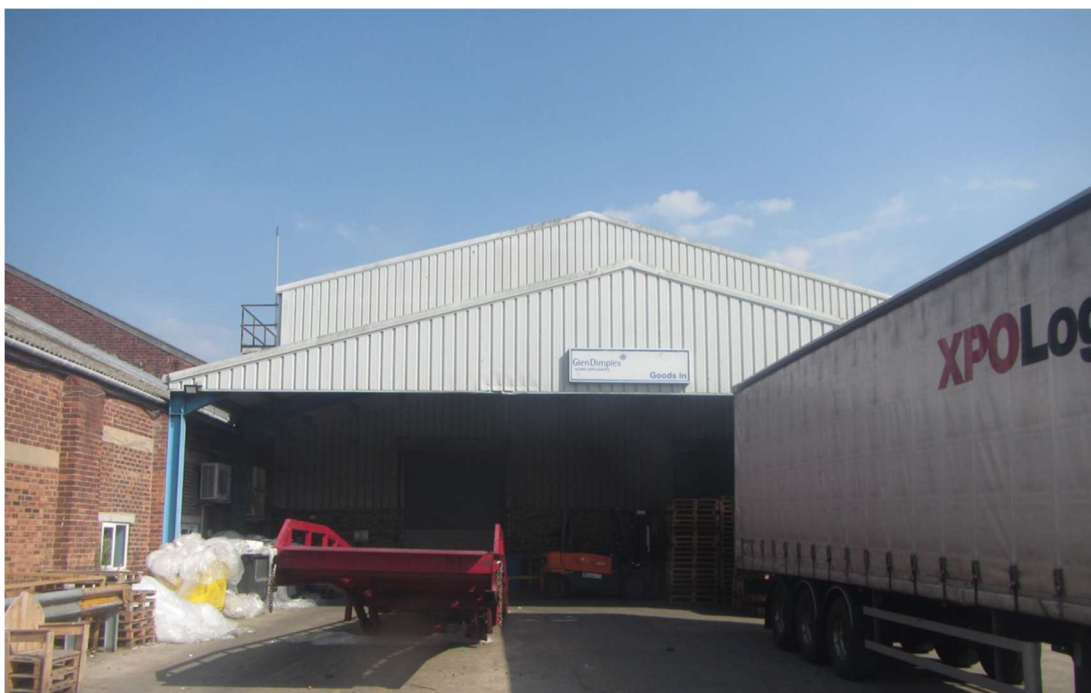
Photograph 5 – A section of Building 1 which is constructed from metal cladding.
