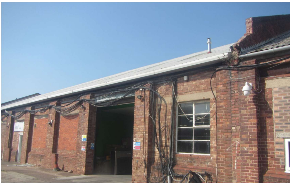
Photograph 4 – Sheet metal roof on Building 1.
