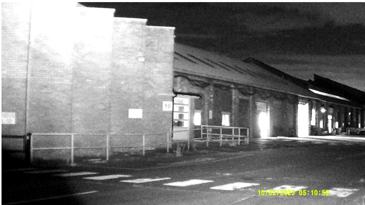
Photograph 24 – Infrared image taken of the southeastern aspect of Building 1 at the darkest point of the survey at 05:10 on 2 nd October 2025.
