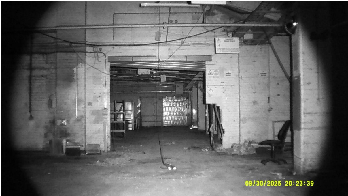
Photograph 19 – Infrared image taken of the northeastern interior of Building 1 at the darkest point of the survey at 20:23 on 30 th September 2025.
