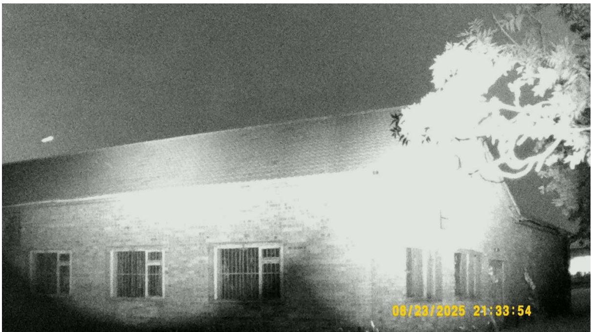
Photograph 2 – Infrared image taken of the southeastern aspect of Building 7 at the darkest point of the survey at 21:33 on 23th August 2025.
