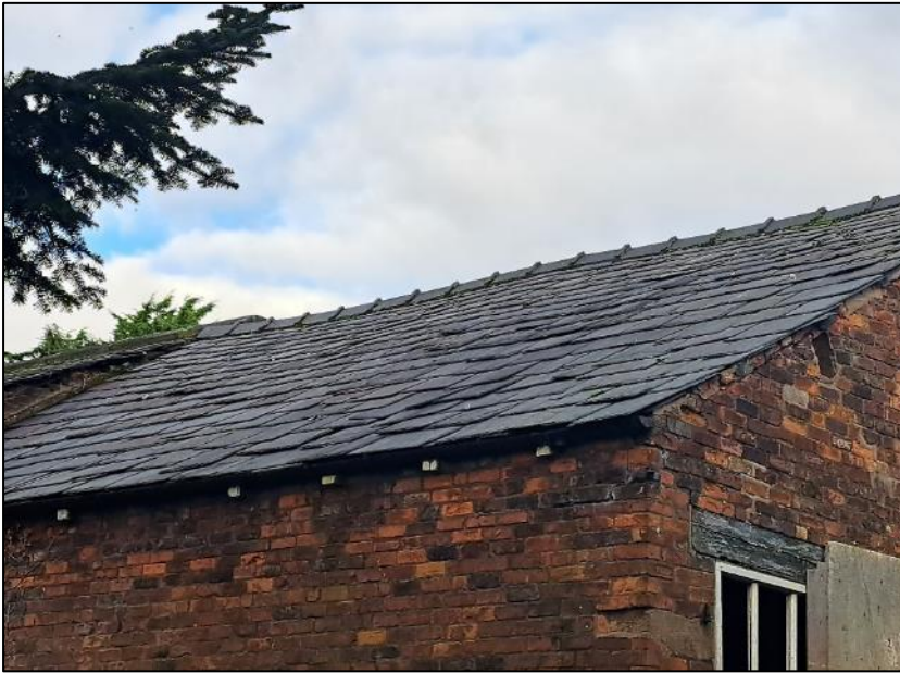
Photograph 14 showing a section of roof on the barn
