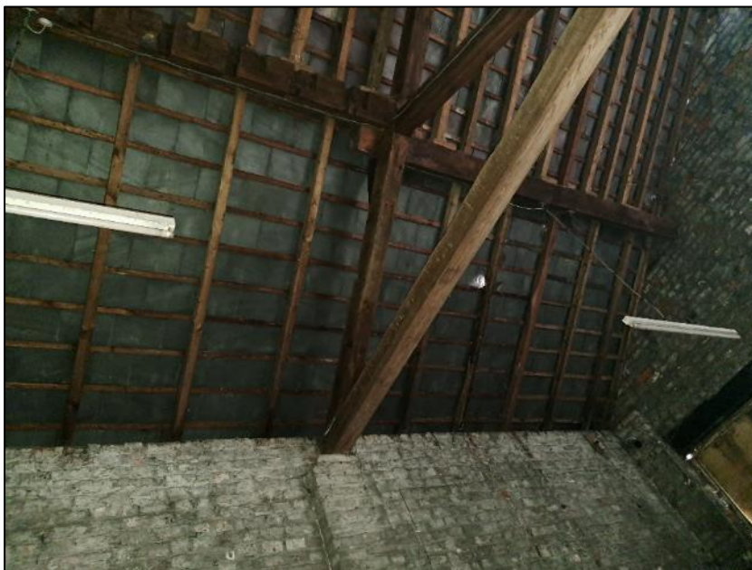
Photograph 19 showing the underside of the roof of the barn
