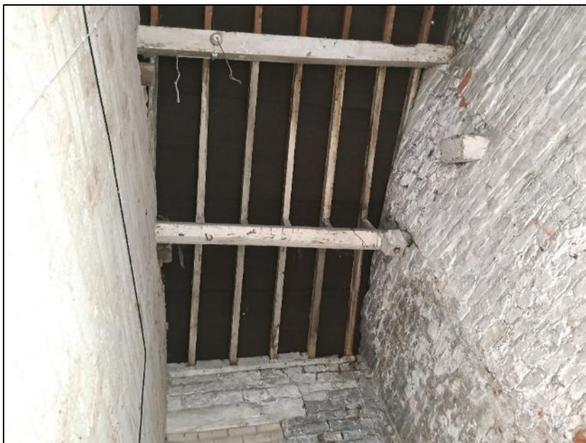
Photograph 22 showing the underside of the roof in the western section of the barn
