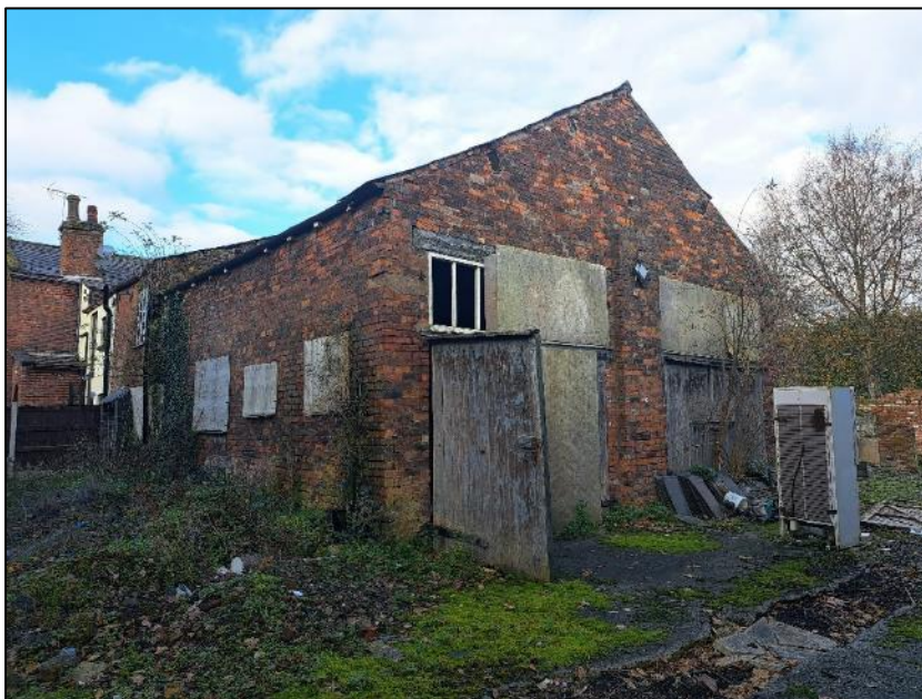
Photograph 11 showing the external masonry of the main barn
