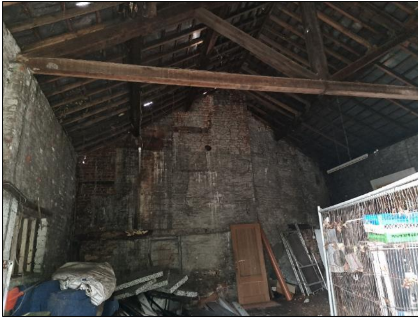
Photograph 18 showing the interior of the barn
