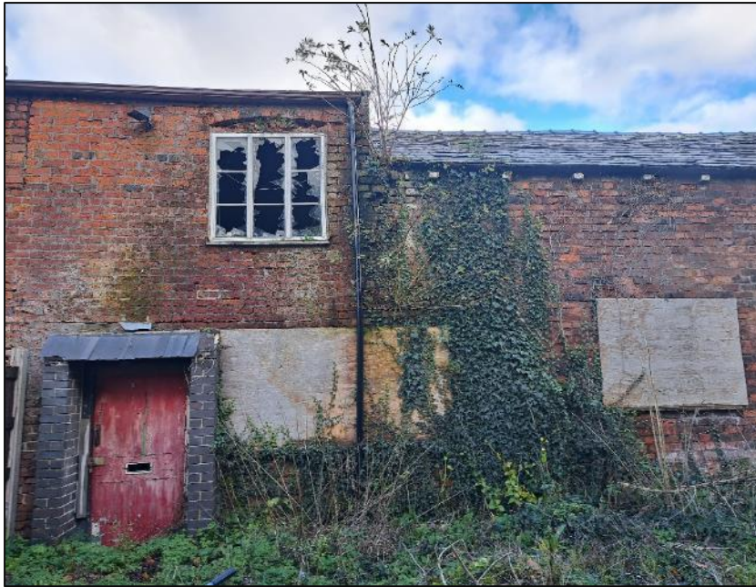
Photograph 16 showing potential access points on the southern elevation of the barn
