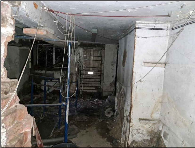
Photograph 20 showing the lower elevation of the western section/room of the barn and open letterbox
