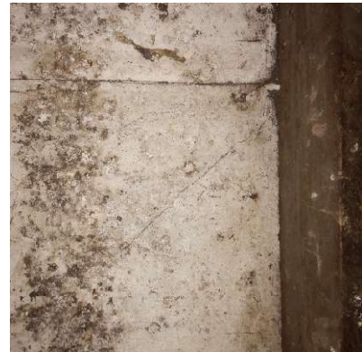
Photos 61-65: Cracked cast fibrous plaster plain panels, exposed hessian and laths within the casts after deterioration of the upper surfaces and patching after a fall of part of a panel.
