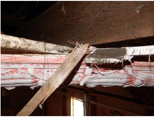
Photos 26 & 27: Broken cast panels in the centre of the first bay expose the nature of the fibrous cast panel and its over skim.
