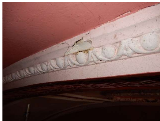
Photos 24 & 25: As well as the impact damage in this bay the adjacent rib has deteriorated with prolonged damp, held against it by guano deposits and requires sections of the fibrous cast replacing.
