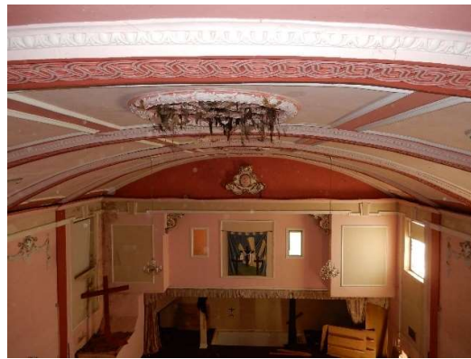
Photos 39 & 40: The plaster ventilation grill in the fourth bay is cracked and requires repair and wiring up.
