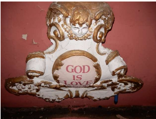
Photos 14, 15 &16: The cartouche, rebranded by the previous church, is hung off the vertical timbers carrying this lath and plaster work. Unfortunately, the top section is badly cracked and needs to be re-secured urgently.
