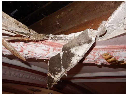
Photos 26 & 27: Broken cast panels in the centre of the first bay expose the nature of the fibrous cast panel and its over skim.
