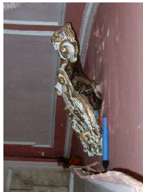
Photos 14, 15 &16: The cartouche, rebranded by the previous church, is hung off the vertical timbers carrying this lath and plaster work. Unfortunately, the top section is badly cracked and needs to be re-secured urgently.
