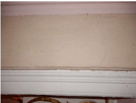
Photos 17-19: The lower edge of the front of the proscenium beam, which is cracked through the plaster on the lath; above the back of the lath and plaster that forms the soffit of the same beam, and a thin coat of gauged lime plaster to the front of the infilled proscenium arch.
