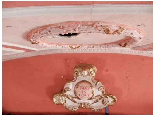
Photos 22 & 23: The first ceiling bay has suffered water and impact damage in the past and has been partly reskimmed or skimmed originally to create a more even arched plain plaster finish coat, but this is in part de-bonding.
