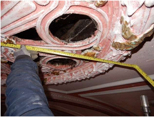
Photos 31 & 32: The plaster ventilation grill in the second bay.
