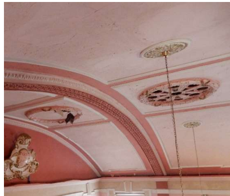
Photos 35 & 36: The first fibrous plaster rib nearest the stage is falling and only supported at its eastern end by the cornice below. The ribs do not appear to have been cast to the correct radius and the unevenness of the curve underlies other visible distress in them.
