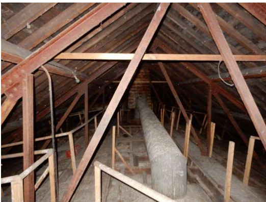
Photos 3 and 4: The ceiling is supported by lightweight fabricated wrought iron trusses, which also support an earlier mechanical ventilation system.
