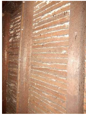
Photos 11, 12 &13: The lath and plaster, with minimal nibs, forming the proscenium arch and the badly warped and deteriorated projecting cornice to the front.
