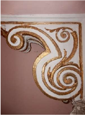
Photos 20 & 21: One of the scrolled corbel console brackets, both of which appear to have been fastened up 90 degrees in the wrong orientation; and the support from above the soffit of the proscenium beam.
