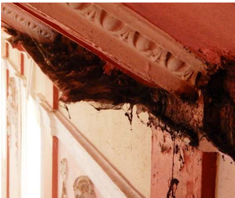
Photos 41 & 42: The almost completely decayed cornice on the western end of the bay; and a cracked edge all the way along the rib between the 4 th and 5 th bay, and the overturning cornice on the east wall.
