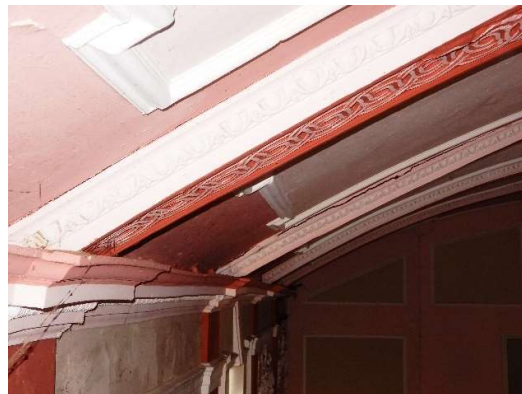
Photos 41 & 42: The almost completely decayed cornice on the western end of the bay; and a cracked edge all the way along the rib between the 4 th and 5 th bay, and the overturning cornice on the east wall.
