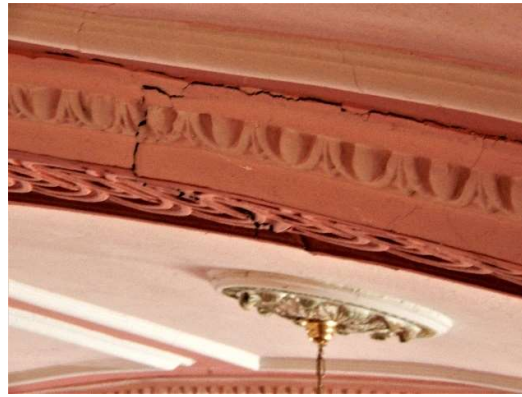
Photos 49 & 50: The failing rib between the 5 th and 4 th bay is clearly visible.
