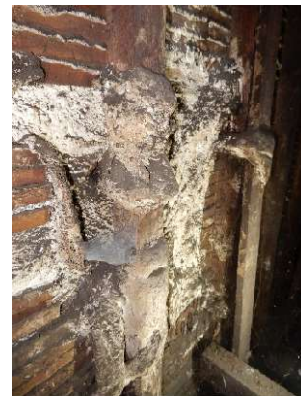
Photos 14, 15 &16: The cartouche, rebranded by the previous church, is hung off the vertical timbers carrying this lath and plaster work. Unfortunately, the top section is badly cracked and needs to be re-secured urgently.
