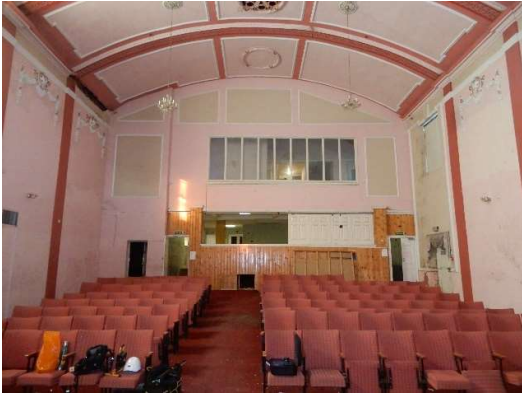
Photos 1 & 2: The barrel vaulted ceiling, decorated with ribs and panel moulding, above the main auditorium space, with a previous open bay beyond the more recent partition at the back and the altered screen/stage area at the front.
