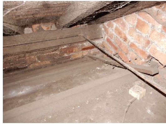
Photos 7 & 8: These ceiling joists sit upon the bottom member of the trusses, and at both ends of the auditorium in pockets formed in the brickwork. Hung off the ceiling trusses are fibrous cast plain panels, which are just nailed on from below. The trusses also carry by unwired fibrous wads, the decorative ceiling ribs which hang directly below them.
