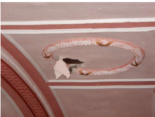
Photos 24 & 25: As well as the impact damage in this bay the adjacent rib has deteriorated with prolonged damp, held against it by guano deposits and requires sections of the fibrous cast replacing.
