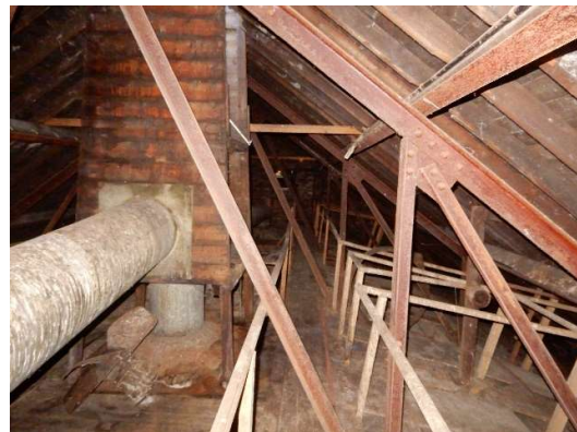
Photos 3 and 4: The ceiling is supported by lightweight fabricated wrought iron trusses, which also support an earlier mechanical ventilation system.
