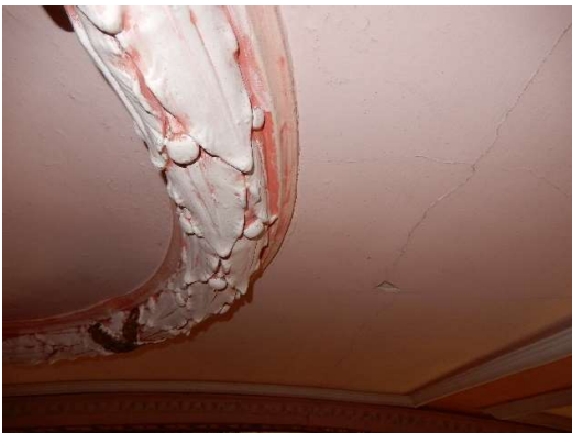
Photos 45-48: Badly water damaged wall and ceiling plaster at the eastern end of the 5 th bay; and cracking and debonding can be seen below the cast ceiling panels.
