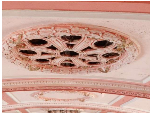
Photos 33 & 34: Whilst the ornamental ventilation cover is in reasonable condition the surrounding plain plaster and the planted on panel mouldings are cracked and there is some debonding of skim plaster.
