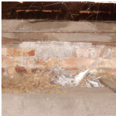
Photos 66-68: Whilst the ceiling void has been cleaned of excessive levels of guano and dead birds, some pockets still remain, reminding us of the extent of weight and moisture previously present in the back of this ceiling.
