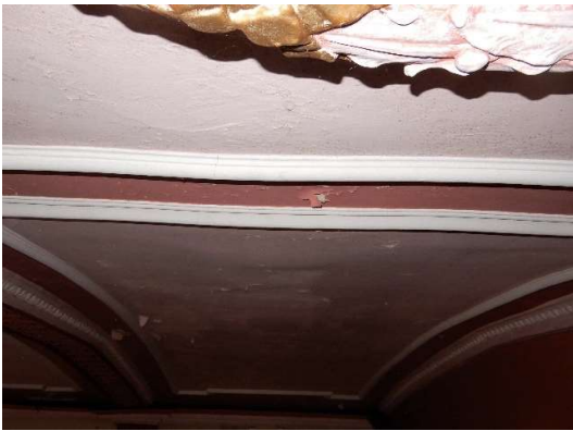
Photos 33 & 34: Whilst the ornamental ventilation cover is in reasonable condition the surrounding plain plaster and the planted on panel mouldings are cracked and there is some debonding of skim plaster.
