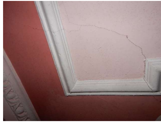
Photos 43 & 44: Debonding and cracked skimmed plaster at the eastern edge of the bay.
