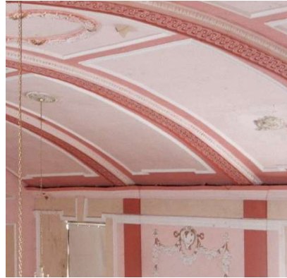
Photos 37 & 38: The distorted and failing cornice can be seen in the first picture; and debonding skim and the area of distress in the centre of the western end of this bay, in the second.
