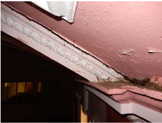
Photos 78 & 79: Damp induced decay of the hessian in the plaster wads carrying the cornices has also meant some ribs may fall soon; and damp in the walls has caused extensive debonding in the wall's plasters, including those carrying the decorative swags.
