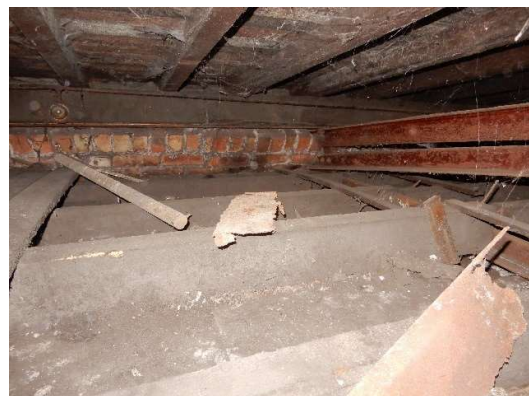
Photos 5 & 6: Running along the length of the ceiling and supported off the tie beams of the steel trusses are substantial ceiling joists
