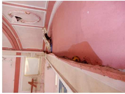
Photos 11, 12 &13: The lath and plaster, with minimal nibs, forming the proscenium arch and the badly warped and deteriorated projecting cornice to the front.
