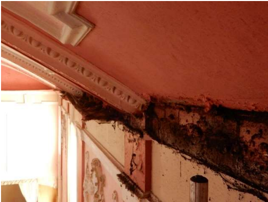
Photos 51 & 52: Water damage has caused the cornice at the western end to be lost and the plaster behind the decorative swags on all the walls has significantly de-bonded from the brick background.
