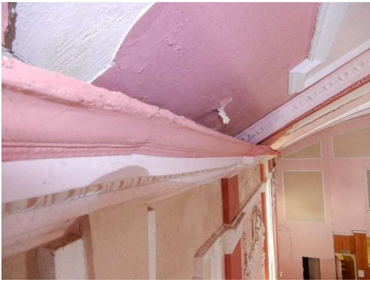
Photos 43 & 44: Debonding and cracked skimmed plaster at the eastern edge of the bay.
