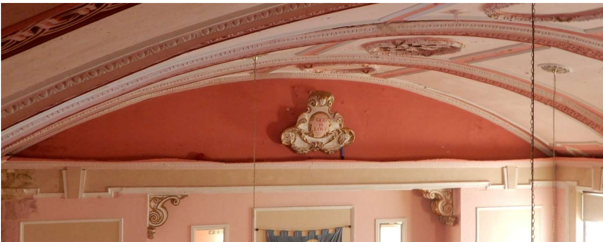
Photo 10: By contrast the enclosed proscenium arch and the proscenium beam below, carried by scroll console brackets, are created with lath and lime plaster gauged with gypsum.
