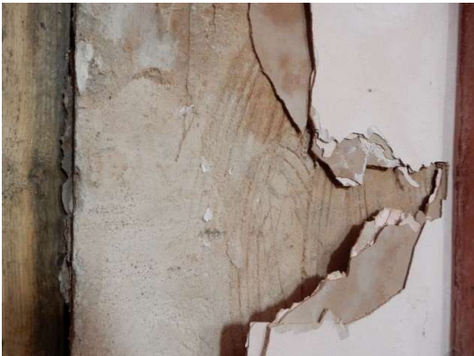
Photo 80: De-bonding modern gypsum based plasters, which has been used to over skim the areas enclosed by and below the balconies, after they were removed.
