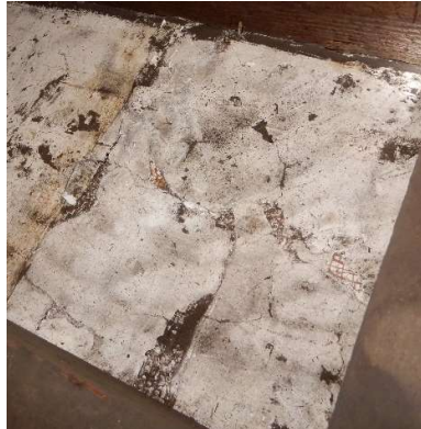
Photos 61-65: Cracked cast fibrous plaster plain panels, exposed hessian and laths within the casts after deterioration of the upper surfaces and patching after a fall of part of a panel.
