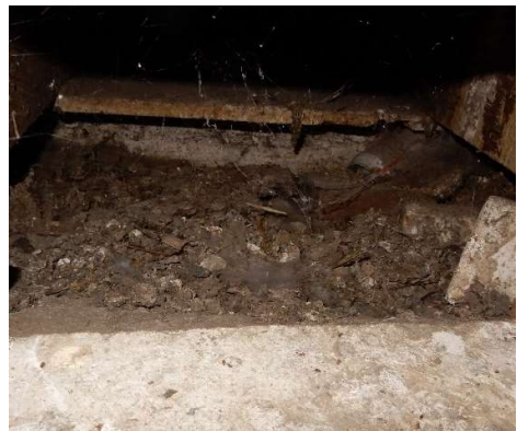
Photos 66-68: Whilst the ceiling void has been cleaned of excessive levels of guano and dead birds, some pockets still remain, reminding us of the extent of weight and moisture previously present in the back of this ceiling.
