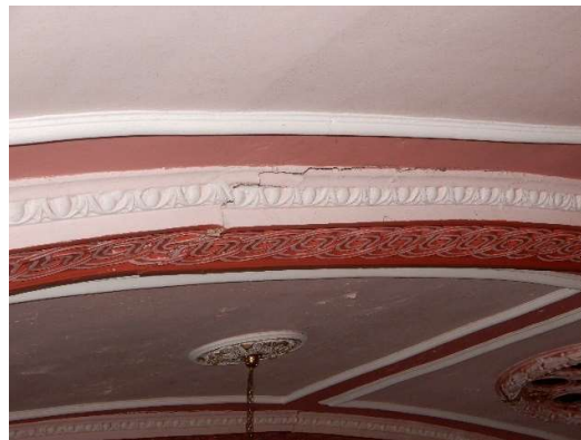
Photos 28 & 29: The ceiling is badly cracked where it meets the front of the proscenium arch; and parts of the first fibrous rib are beginning to fall.
