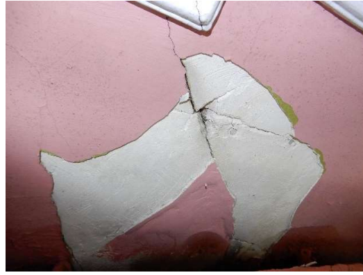
Photos 76 & 77: The cast plaster panels are carried off ceiling joists parallel but not touching the external brickwork, has reduced the amount of damage at the ceiling edges; damp and impact damage however has still caused debonding of the skim found under some of the boards.
