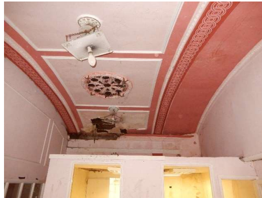
Photos 53 and 54: The distressed eastern third of the 6 th bay; and the collapsed western end, although the plaster ventilation grill is in reasonable condition.
