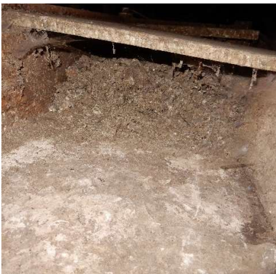
Photos 66-68: Whilst the ceiling void has been cleaned of excessive levels of guano and dead birds, some pockets still remain, reminding us of the extent of weight and moisture previously present in the back of this ceiling.
