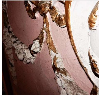
Photos 51 & 52: Water damage has caused the cornice at the western end to be lost and the plaster behind the decorative swags on all the walls has significantly de-bonded from the brick background.
