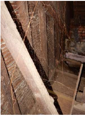
Photos 11, 12 &13: The lath and plaster, with minimal nibs, forming the proscenium arch and the badly warped and deteriorated projecting cornice to the front.
