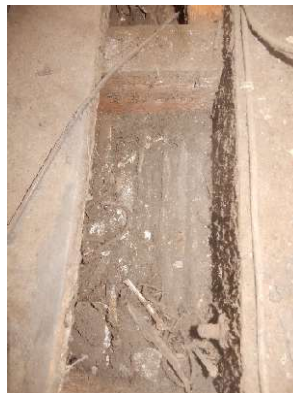
Photos 17-19: The lower edge of the front of the proscenium beam, which is cracked through the plaster on the lath; above the back of the lath and plaster that forms the soffit of the same beam, and a thin coat of gauged lime plaster to the front of the infilled proscenium arch.
