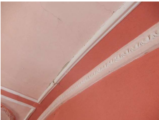
Photos 28 & 29: The ceiling is badly cracked where it meets the front of the proscenium arch; and parts of the first fibrous rib are beginning to fall.
