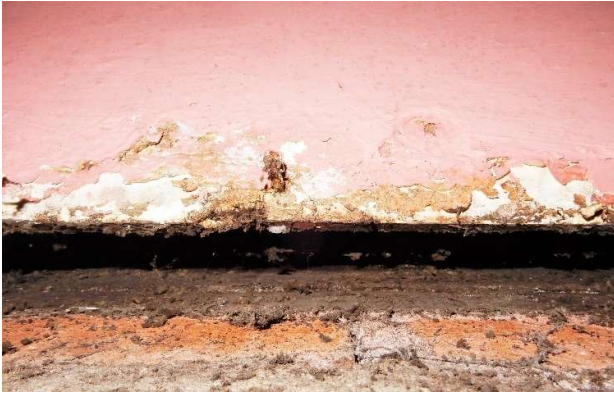
Photos 76 & 77: The cast plaster panels are carried off ceiling joists parallel but not touching the external brickwork, has reduced the amount of damage at the ceiling edges; damp and impact damage however has still caused debonding of the skim found under some of the boards.
