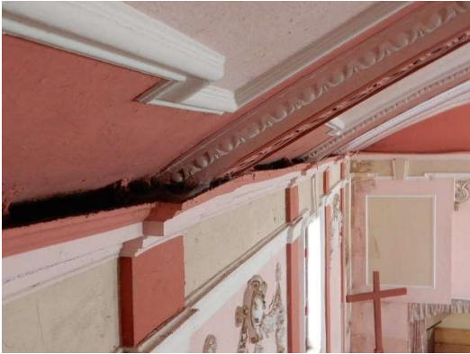
Photos 37 & 38: The distorted and failing cornice can be seen in the first picture; and debonding skim and the area of distress in the centre of the western end of this bay, in the second.
