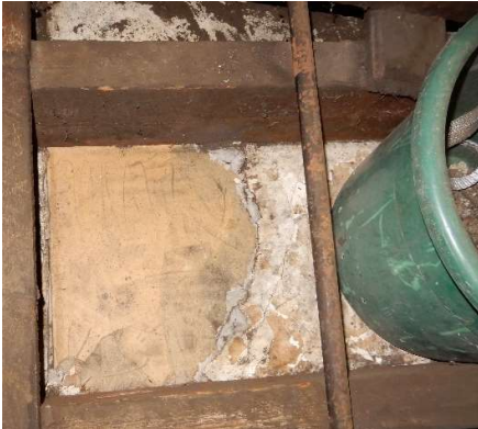
Photos 61-65: Cracked cast fibrous plaster plain panels, exposed hessian and laths within the casts after deterioration of the upper surfaces and patching after a fall of part of a panel.
