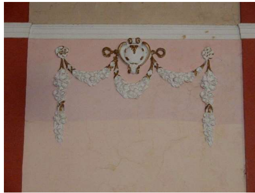
Photos 78 & 79: Damp induced decay of the hessian in the plaster wads carrying the cornices has also meant some ribs may fall soon; and damp in the walls has caused extensive debonding in the wall's plasters, including those carrying the decorative swags.
