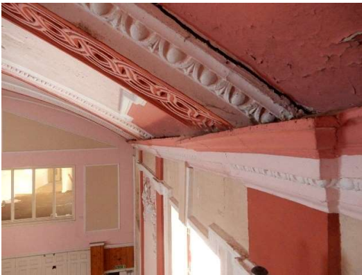
Photos 35 & 36: The first fibrous plaster rib nearest the stage is falling and only supported at its eastern end by the cornice below. The ribs do not appear to have been cast to the correct radius and the unevenness of the curve underlies other visible distress in them.
