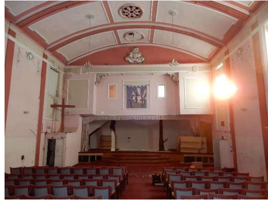
Photos 1 & 2: The barrel vaulted ceiling, decorated with ribs and panel moulding, above the main auditorium space, with a previous open bay beyond the more recent partition at the back and the altered screen/stage area at the front.
