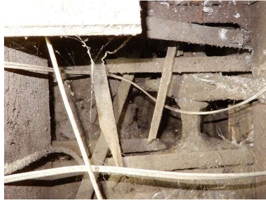
Photos 20 & 21: One of the scrolled corbel console brackets, both of which appear to have been fastened up 90 degrees in the wrong orientation; and the support from above the soffit of the proscenium beam.
