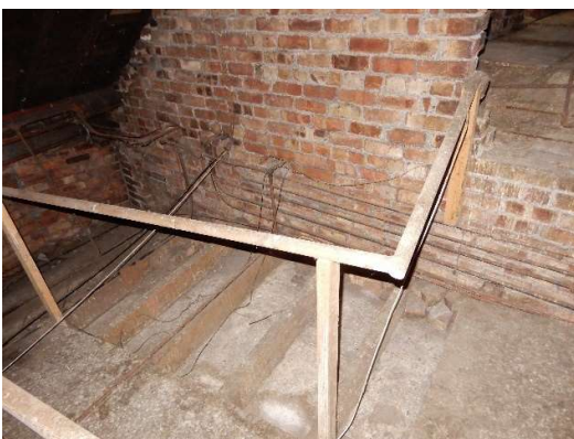
Photo 60: The extra width of the bay at the eastern end has been formed using lath and plaster.
