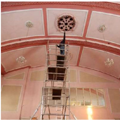
Photos 39 & 40: The plaster ventilation grill in the fourth bay is cracked and requires repair and wiring up.
