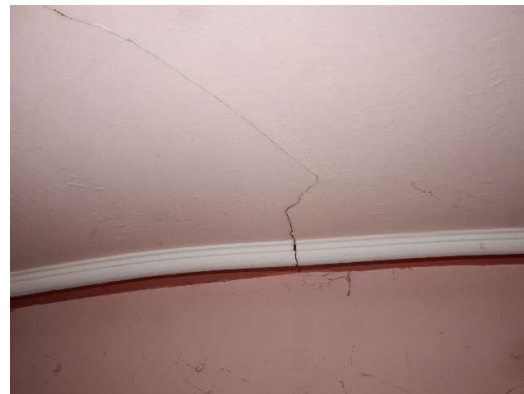
Photos 45-48: Badly water damaged wall and ceiling plaster at the eastern end of the 5 th bay; and cracking and debonding can be seen below the cast ceiling panels.
