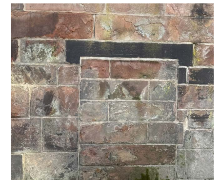
Rich red darker Lintels - Blue Bell Lane
