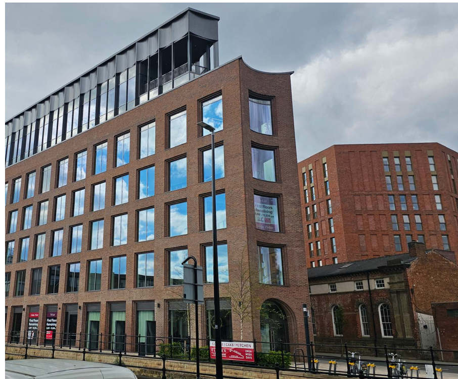
Figure 1.23: Globe Point, Leeds by Feilden Clegg Bradley
