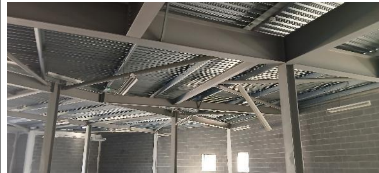
Interior of B2
