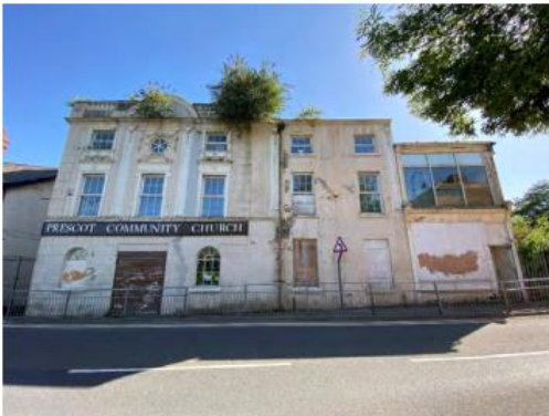
The building as viewed from the road
