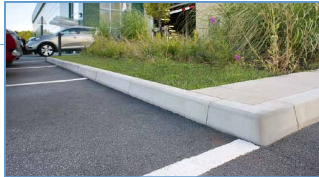
Black permeable tarmac Parking areas defined with thermoplastic paint line markings
