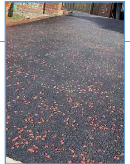
Black permeable tarmac with red chippings
