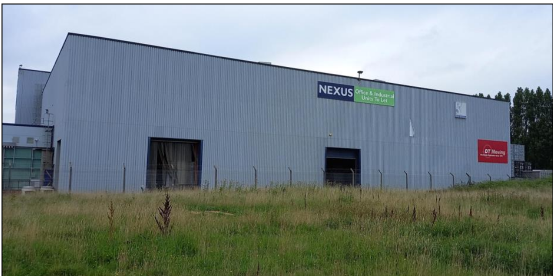
Photograph 4: Northern Section of off-site building
