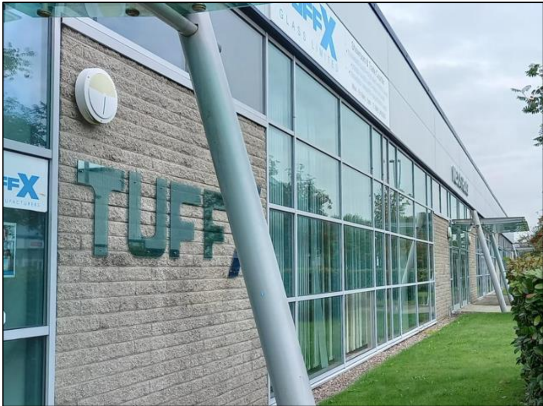
Photograph 3: Southern section of offsite building
