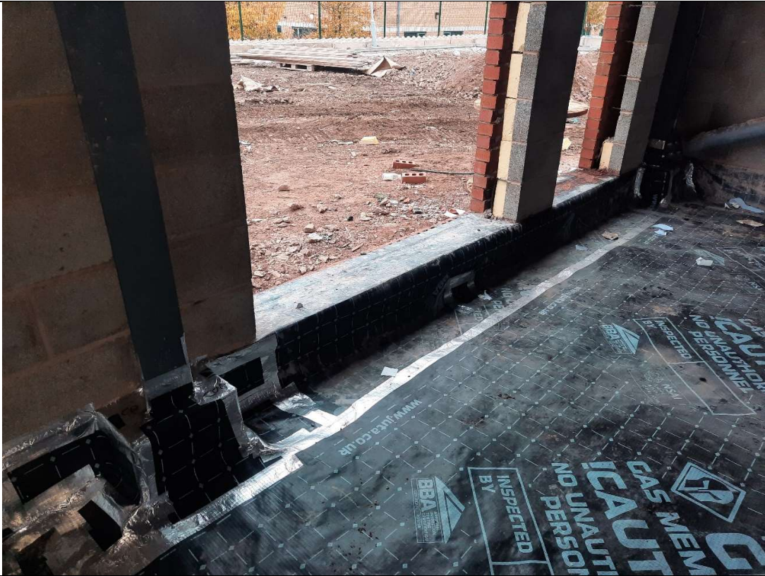
Photo 3 – Sealed membrane DPC section on first stage of inspection.
