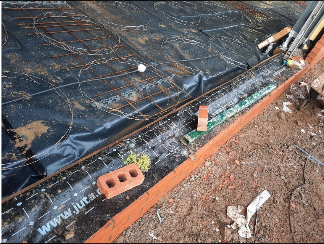
Photo 9 – Sealed DPC membrane section on 3 rd stage of inspection.
