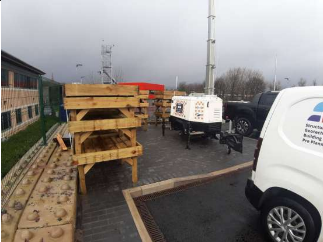
Photo 1 – Showing completed hardstanding in the north east corner of the site (formerly proposed as soft landscaping).
