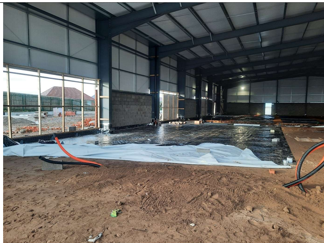
Photo 5 – General condition of membrane on 2nd stage of inspection.
