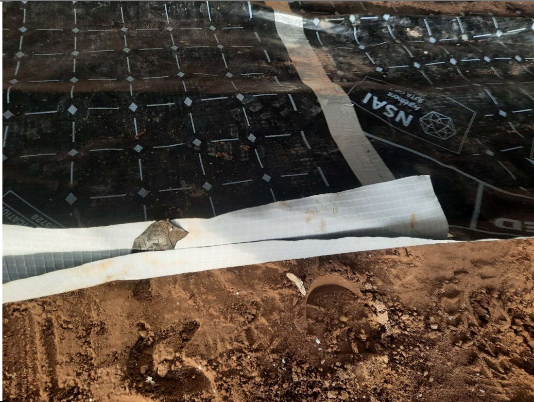
Photo 7 – Membrane joint sealed with butyl tape and jointing tape on 2 nd stage of inspection.
