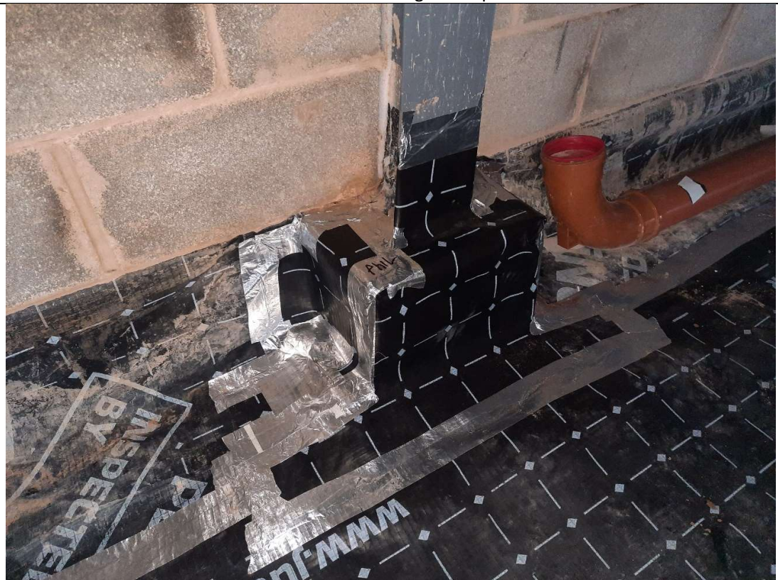
Photo 2 – Membrane sealed to gable column on first stage of inspection.
