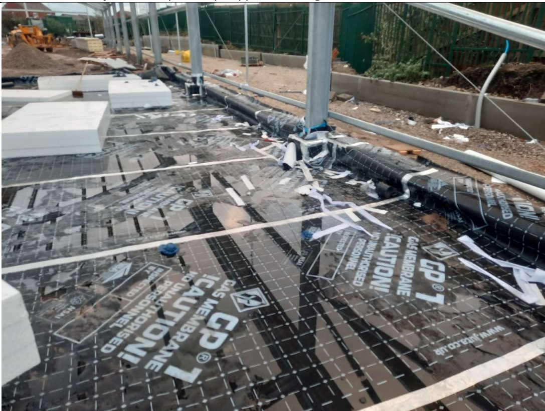
Photo 4 – General condition of the gas membrane
