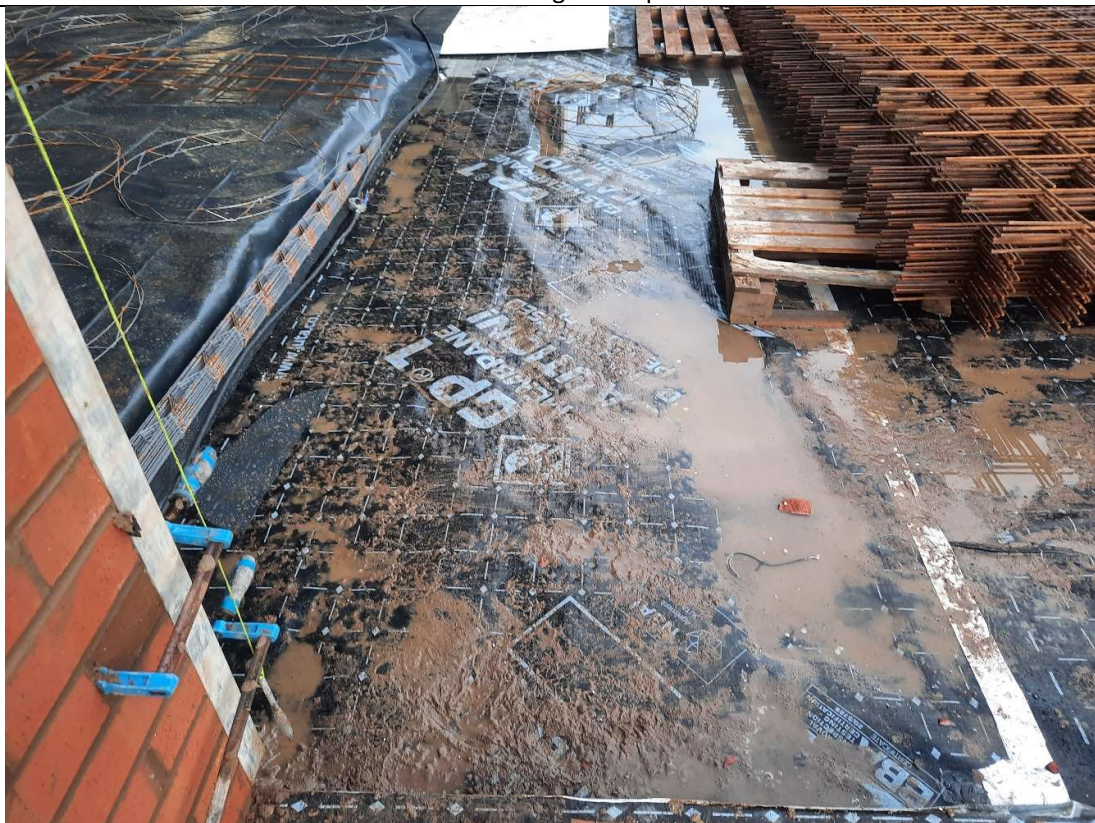
Photo 10 – General condition of membrane on 3 rd stage of inspection.
