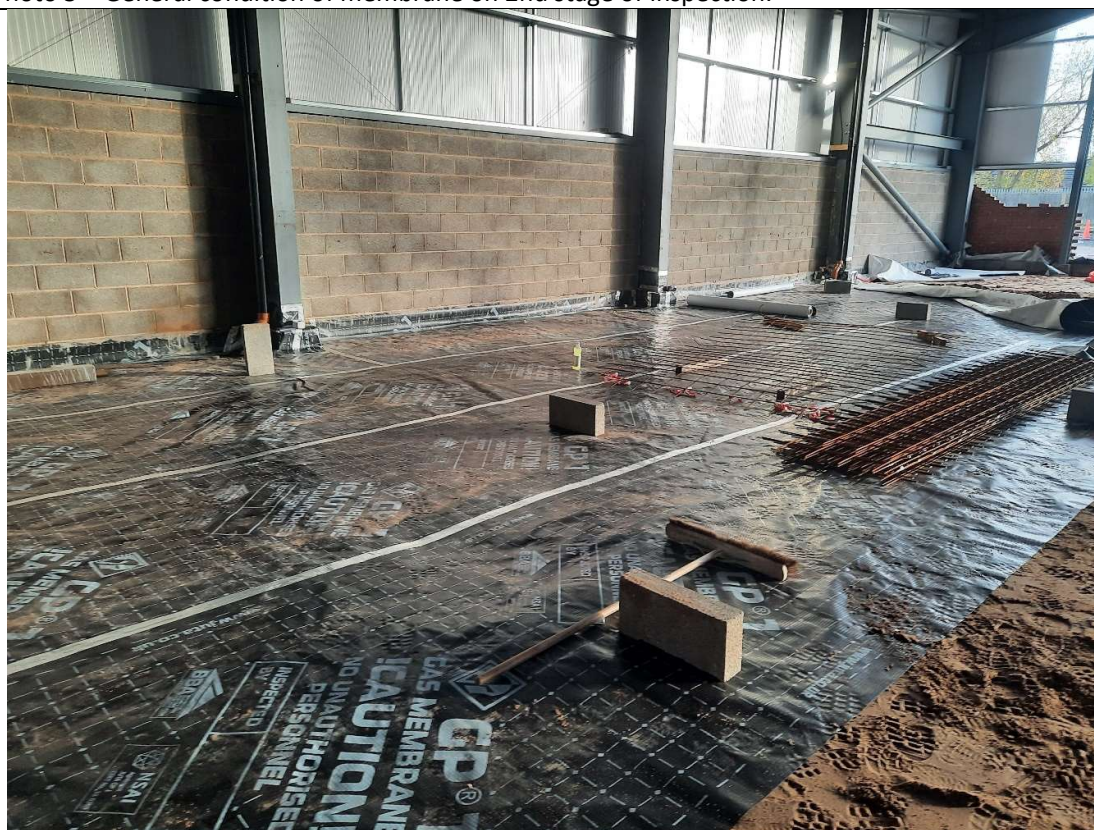
Photo 6 – General condition of membrane on 2nd stage of inspection.
