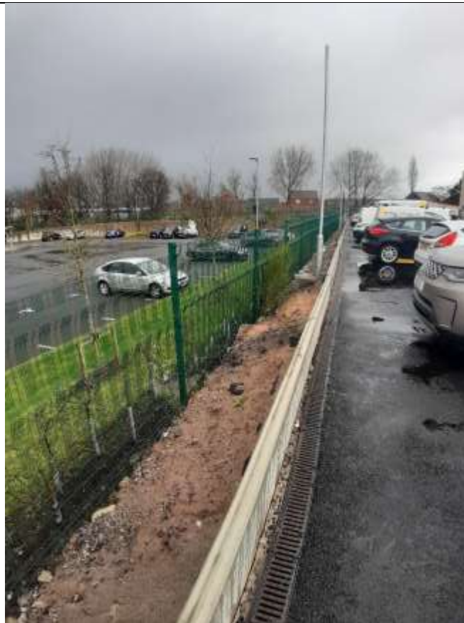
Photo 4 – Showing the northern boundary of the site which is due to be covered by hardstanding.
