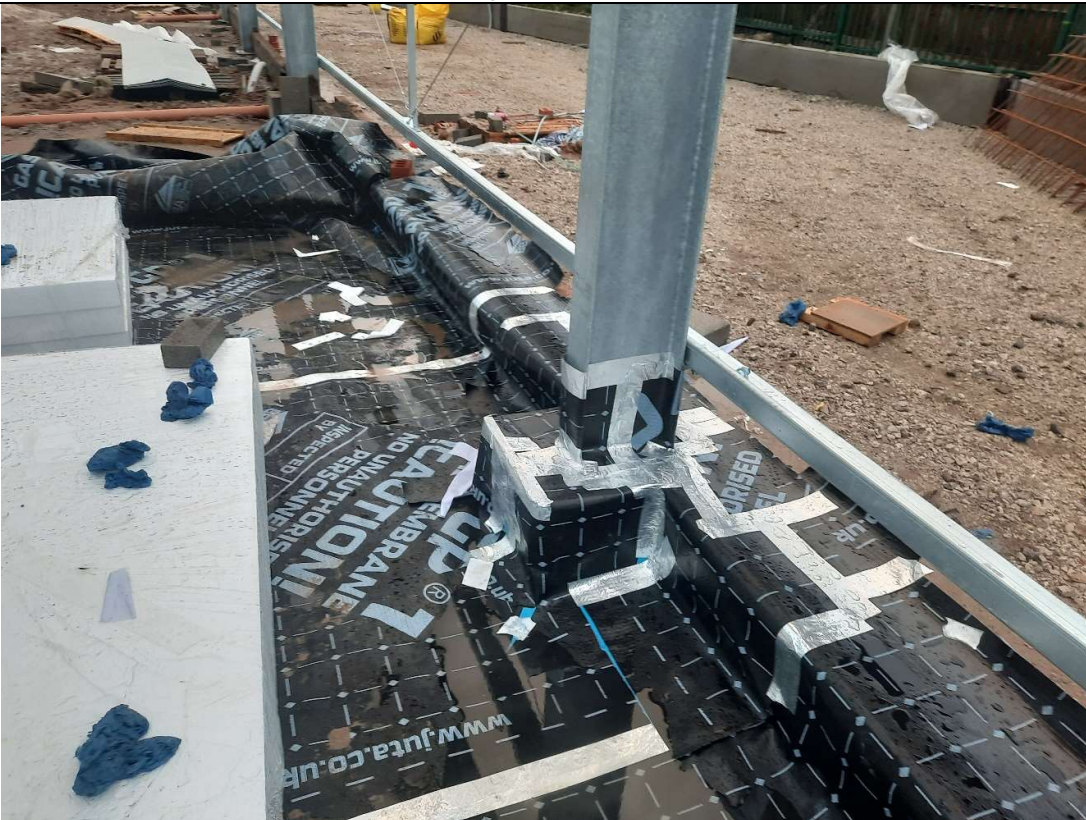
Photo 2 – Sealed column sections and DPC sections of gas membrane.
