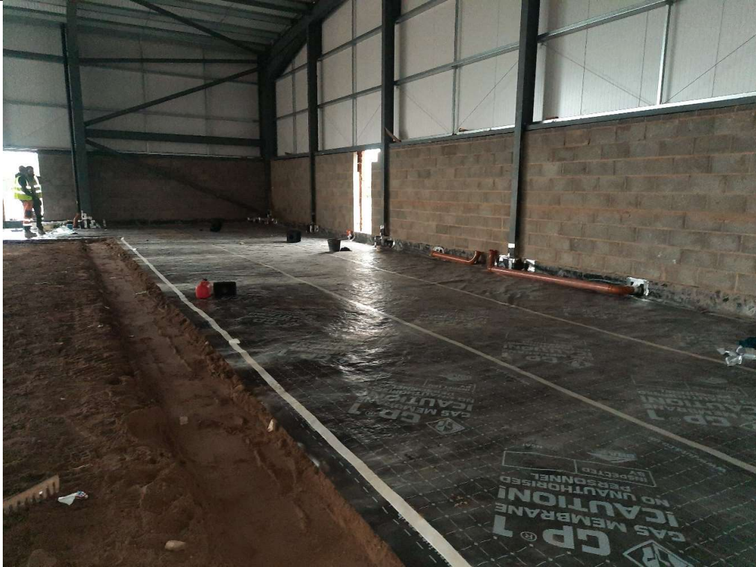
Photo 1 – General condition of membrane on first stage of inspection.
