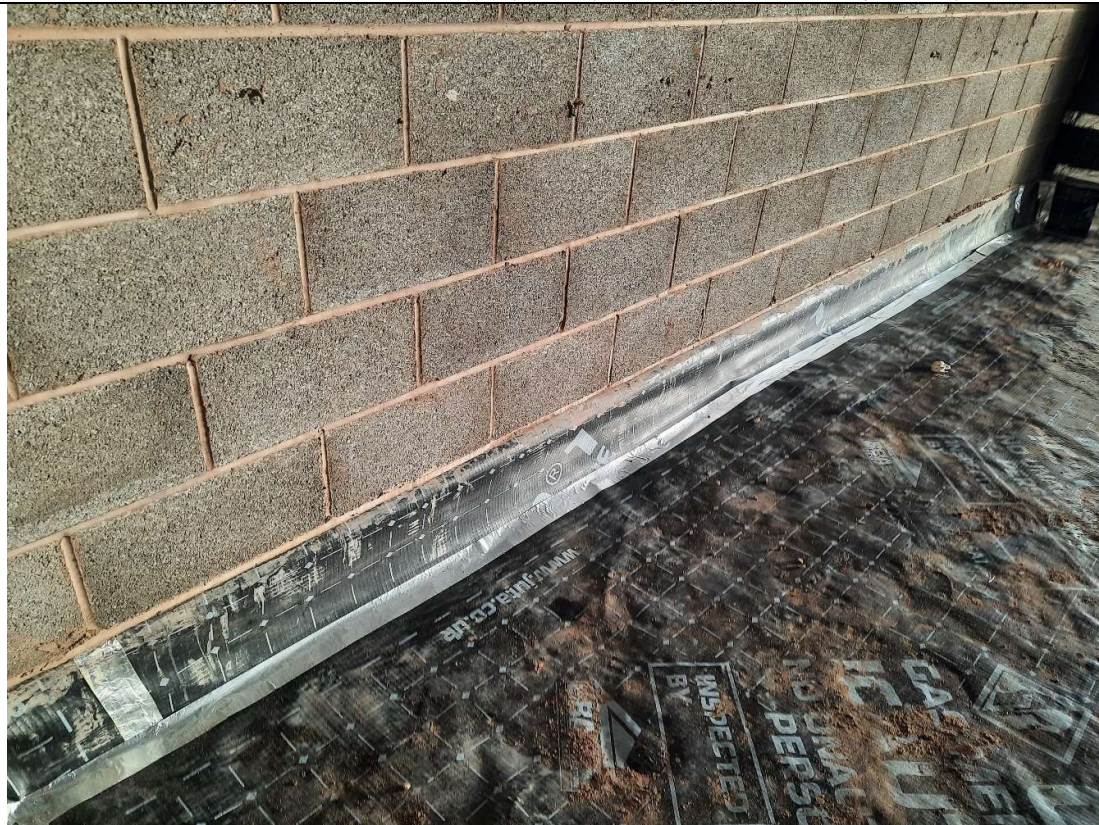
Photo 8 – Sealed DPC membrane section on 2 nd stage of inspection.
