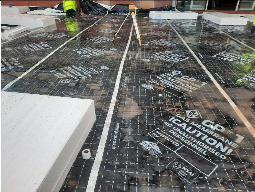
Photo 1 – General condition of the Juta GP-1 gas membrane.
