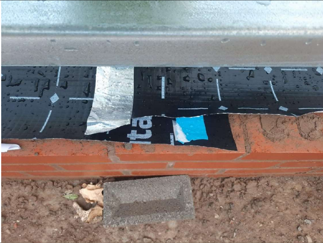
Photo 3 – Sufficient joint overlap and tape application on gas membrane.
