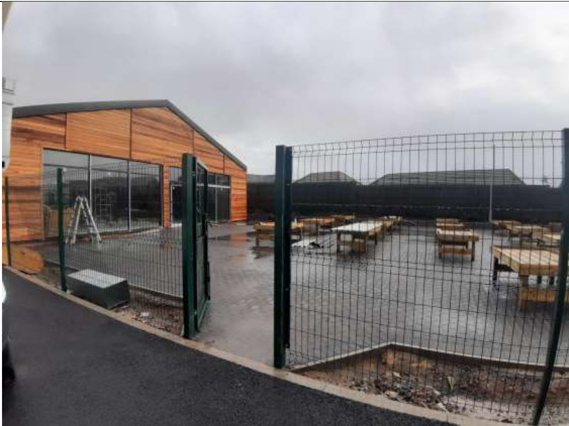
Photo 3 – Showing completed hardstanding in the south west corner of the site (formerly proposed as soft landscaping)
