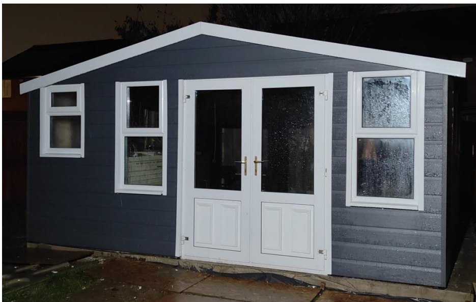
Garden Room Current progress photograph.
