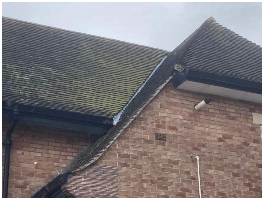
Photograph 4 - Damaged hip tile at the south-east corner of the building (Target Note 2)
