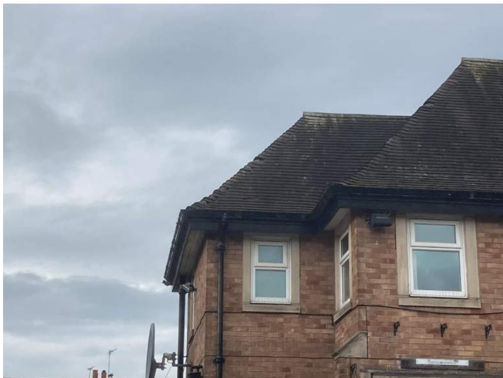
Photograph 7 - Damaged hip tiles at Target Note 3
