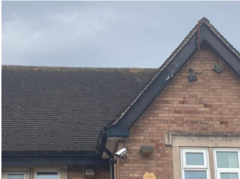
Photograph 7 - Damaged hip tiles at Target Note 3
