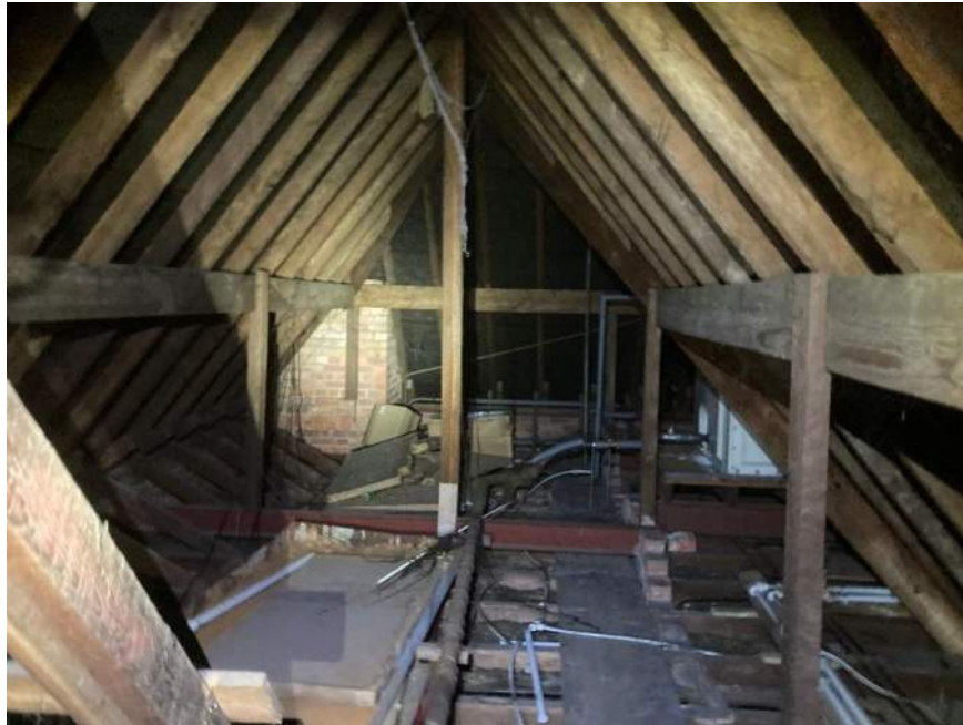
Photograph 7 - Interior of the loft space
