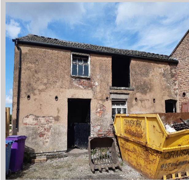
Photograph 9: Stone Barn B (eastern aspect)
