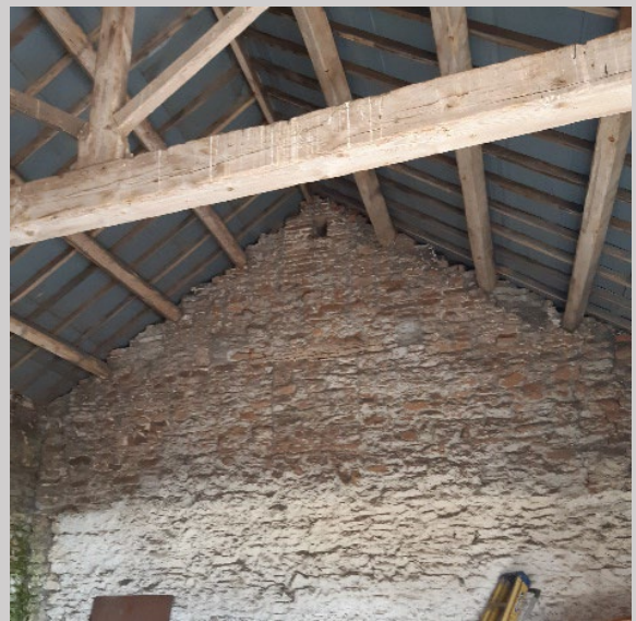
Photograph 4: Stone Barn A roof cavities
