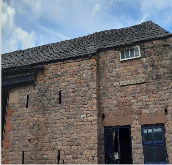
Photograph 1: Stone Barn A front view (eastern aspect)
