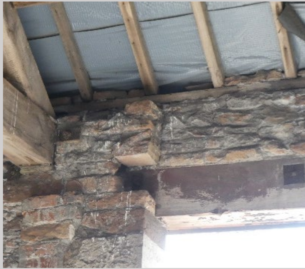
Photograph 5: Stone Barn A roof lining (BRM)
