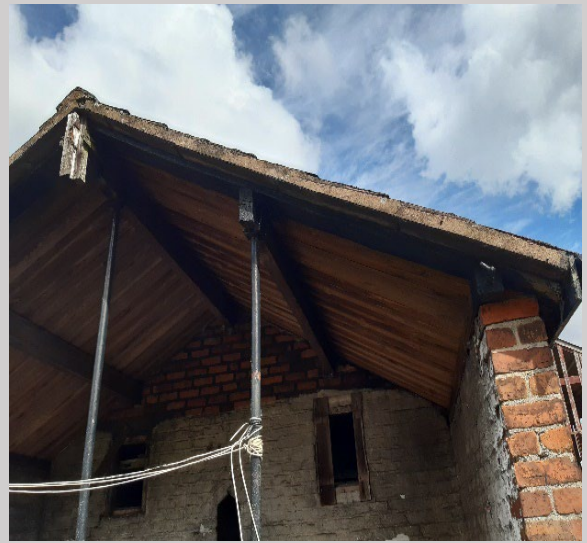
Photograph 18: Piggery pig and bird entrances (southern aspect)
