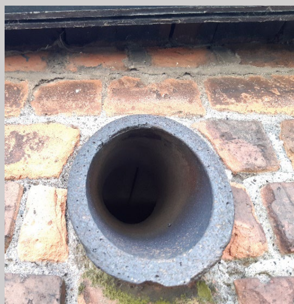
Photograph 16: Piggery ventilation tubes
