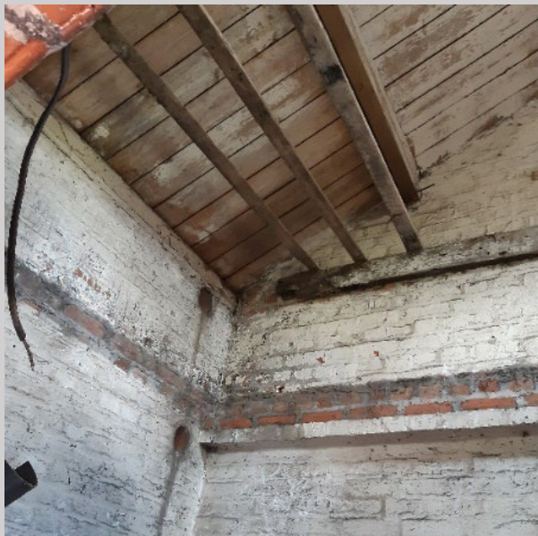
Photograph 19: Piggery timber sarking lining roof
